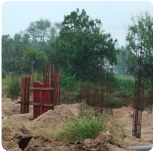
VILLA NO: 1 Pedestals Completed
