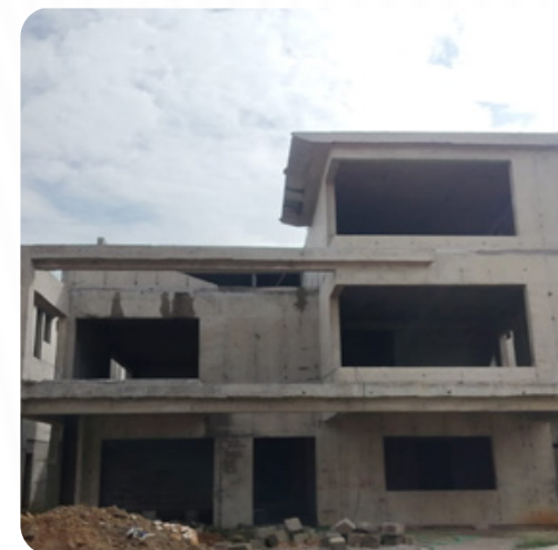
VILLA NO: 151 Block Work Completed
