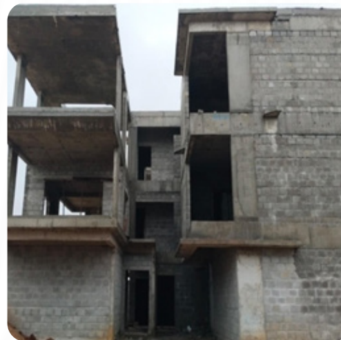
VILLA NO: 35 Brick Work Completed
