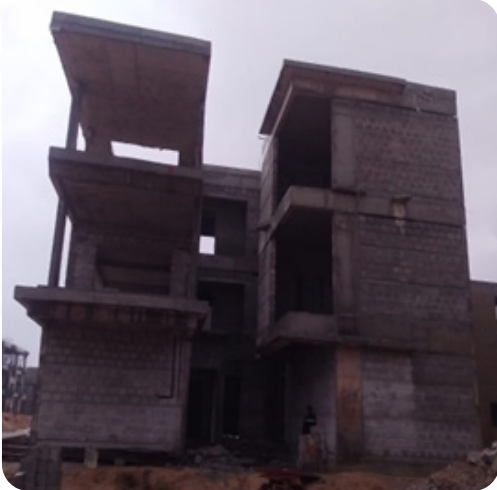
VILLA NO: 79 Brick Work Completed
