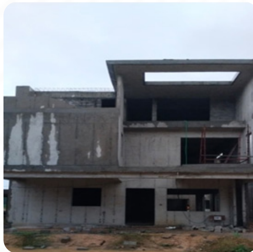
VILLA NO: 125 Block Work Completed
