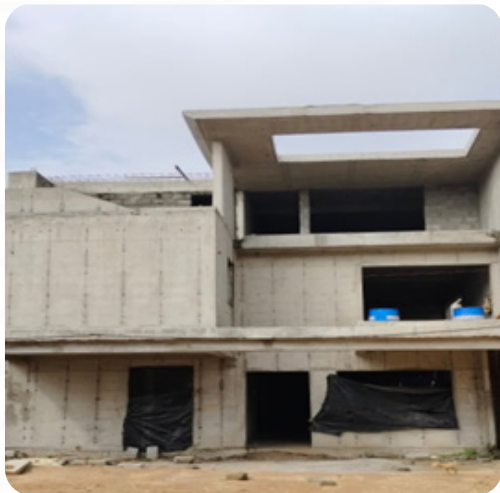
VILLA NO: 156 Block Work Completed
