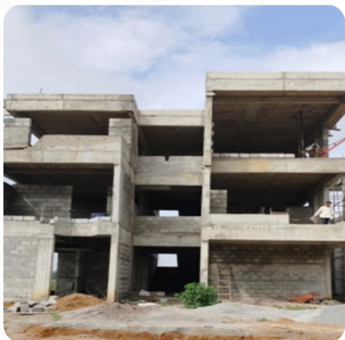
VILLA NO: 180 Brick Work Completed
