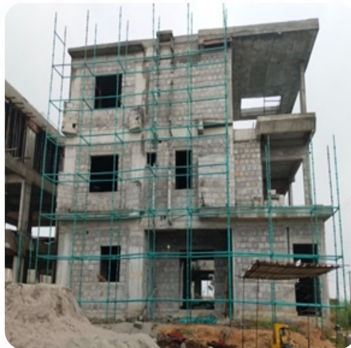
VILLA NO: 42 Brick Work Completed
