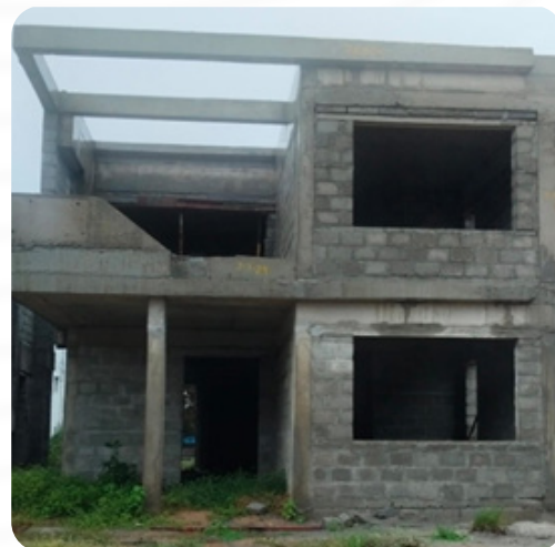
VILLA NO: 5 Brick Work Completed
