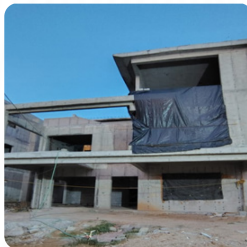
VILLA NO: 174 Block Work Completed
