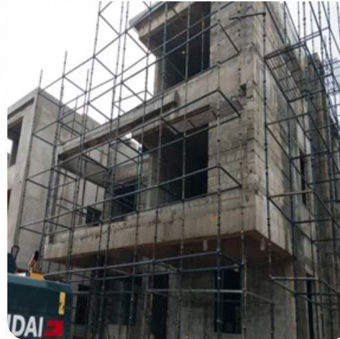
VILLA NO: 47 Slab Completed
