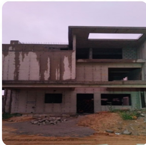
VILLA NO: 133 Block Work Completed
