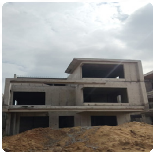
VILLA NO: 144 Block Work Completed
