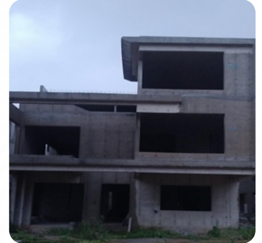
VILLA NO: 83 Block Work Completed
