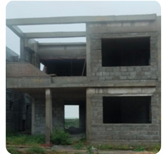
VILLA NO: 4 Brick Work Completed
