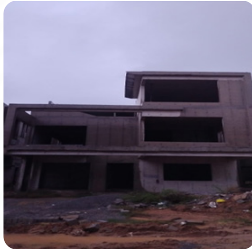
VILLA NO: 89 Block Work Completed
