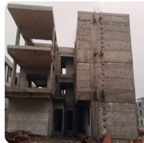
VILLA NO: 115 Brick Work Completed
