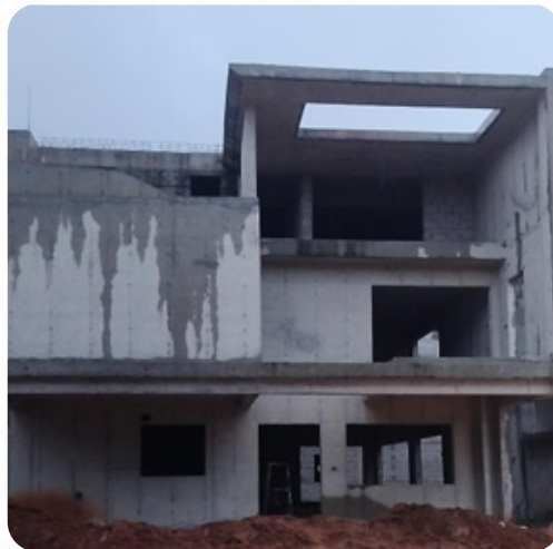
VILLA NO: 75 Block Work Completed
