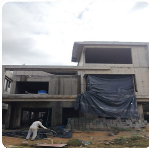
VILLA NO: 177 Block Work Complete
