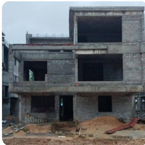
VILLA NO: 50 Brick Work Completed
