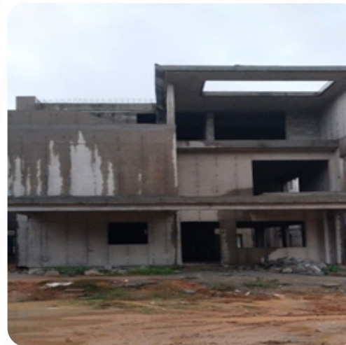
VILLA NO: 126 Block Work Completed
