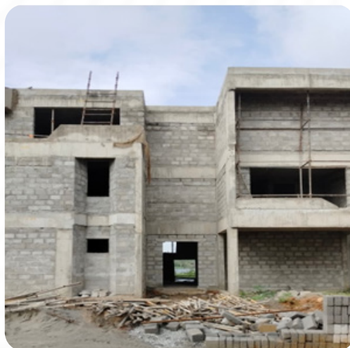
VILLA NO: 181 Brick Work Completed
