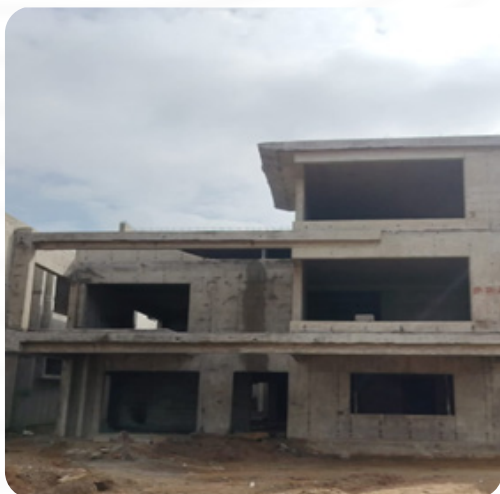
VILLA NO: 148 Block Work Completed
