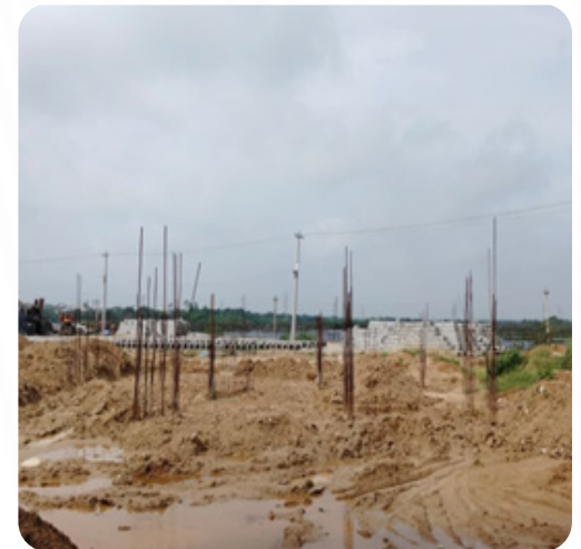
VILLA NO: 167 Plinth Work Completed
