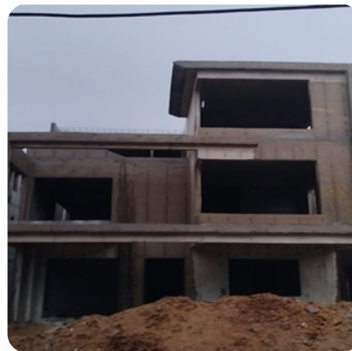
VILLA NO: 118 Block Work Completed
