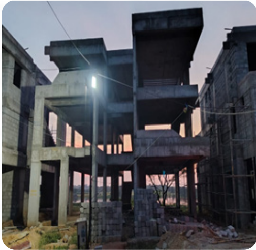
VILLA NO: 184 Slabs Completed
