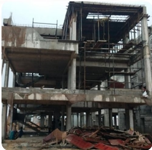
VILLA NO: 41 Slabs Completed
