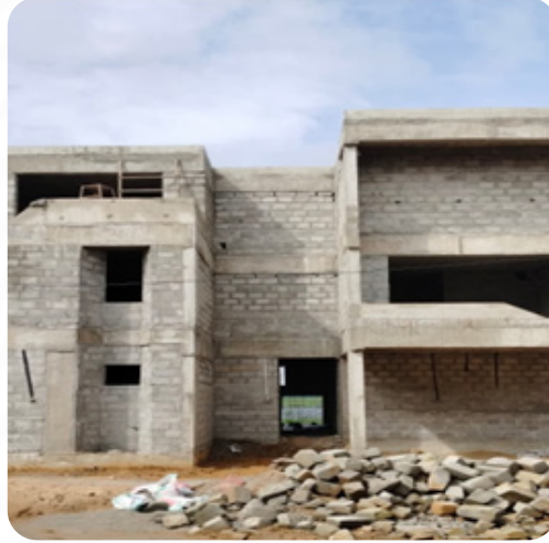
VILLA NO: 185 Brick Work Completed
