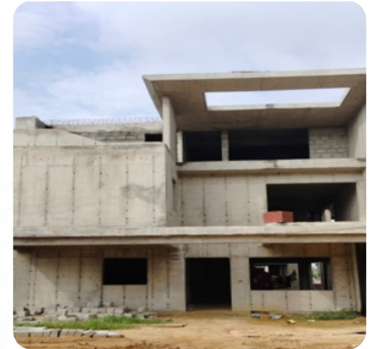
VILLA NO: 155 Block Work Completed
