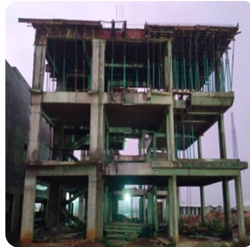
VILLA NO: 138 Slab Work Completed
