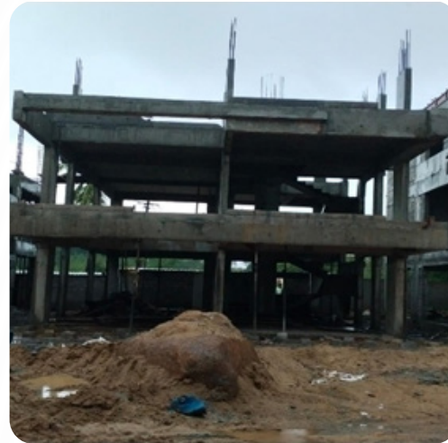
VILLA NO: 56 FF Slab Completed
