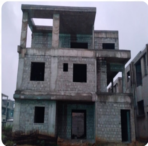
VILLA NO: 132 Brick Work Completed
