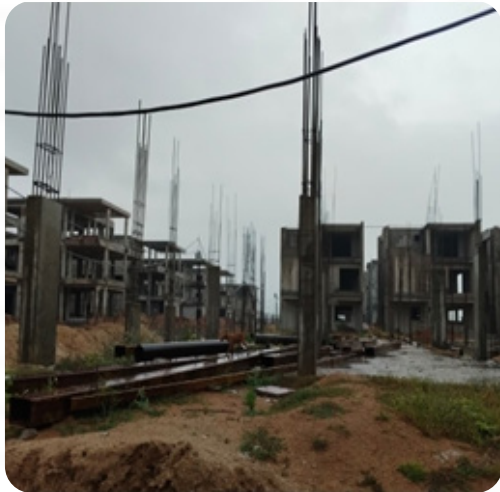
VILLA NO: 12 Columns Completed
