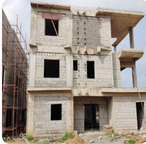
VILLA NO: 161 Brick Work Completed
