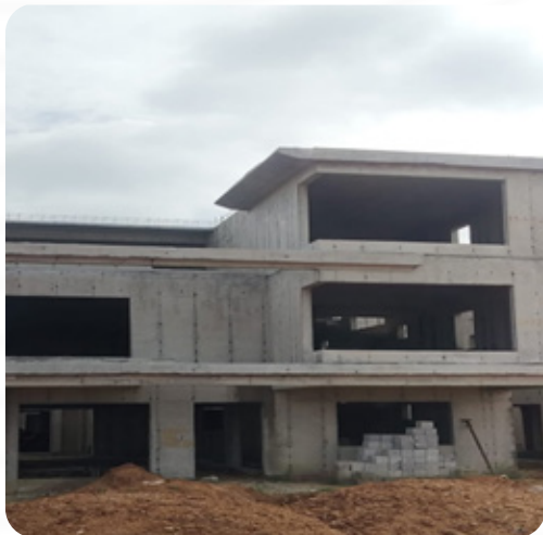
VILLA NO: 140 Block Work Completed
