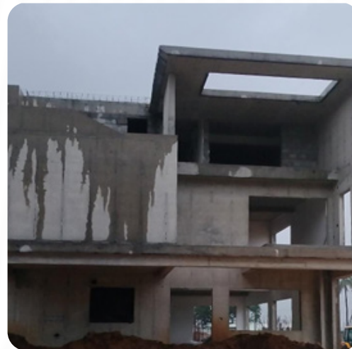
VILLA NO: 76 Block Work Completed
