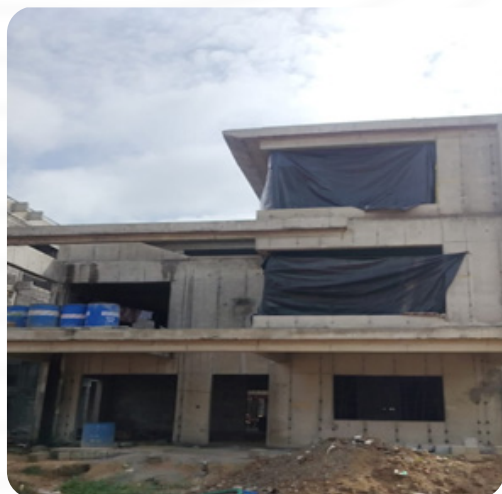
VILLA NO: 172 Block Work Completed
