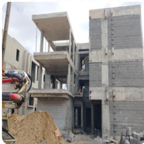
VILLA NO: 145 Brick Work Completed
