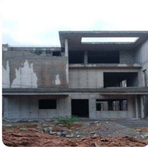
VILLA NO: 129 Block Work Completed
