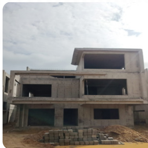
VILLA NO: 150 Block Work Completed
