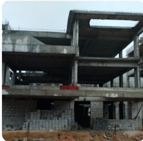
VILLA NO: 26 Slab Work Completed
