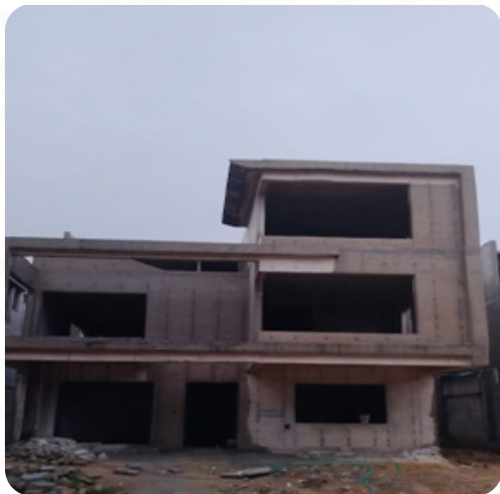
VILLA NO: 112 Block Work Completed
