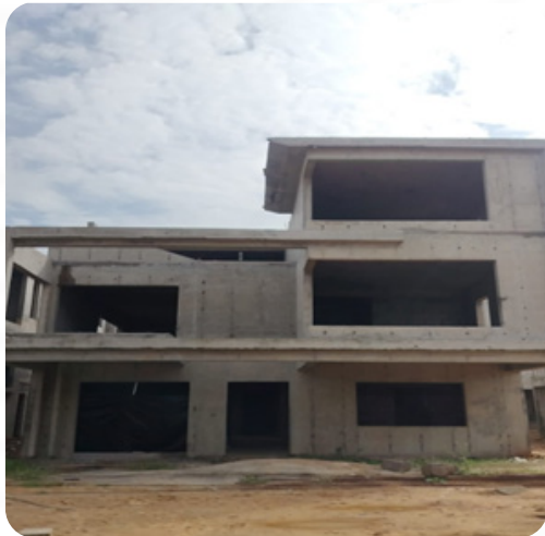
VILLA NO: 152 (Structure Completed)
