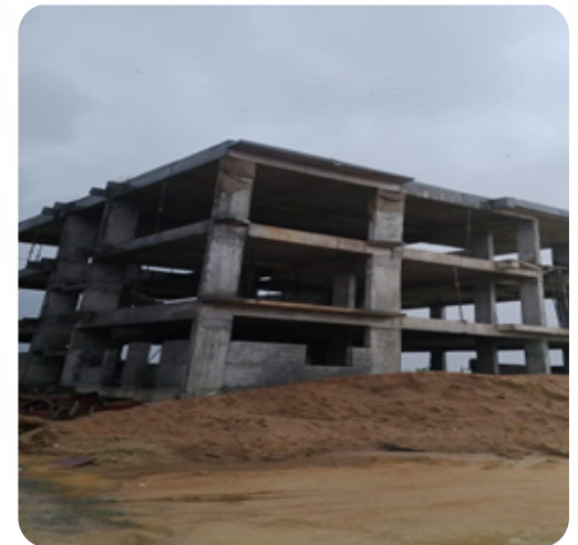
VILLA NO: 77 Block Work Completed
