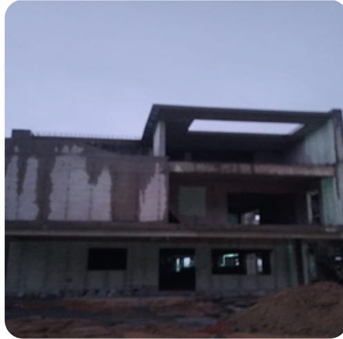
VILLA NO: 137 Block Work Completed
