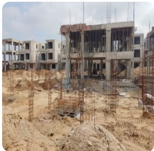
VILLA NO: 168 Plinth Work Completed
