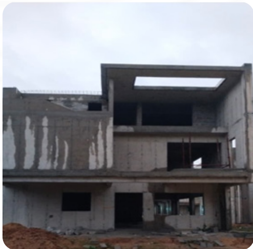
VILLA NO: 124 Block Work Completed
