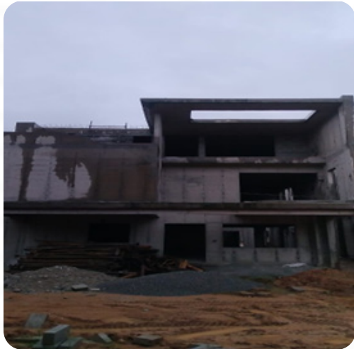
VILLA NO: 96 Block Work Completed
