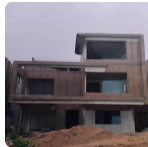
VILLA NO: 119 Block Work Completed
