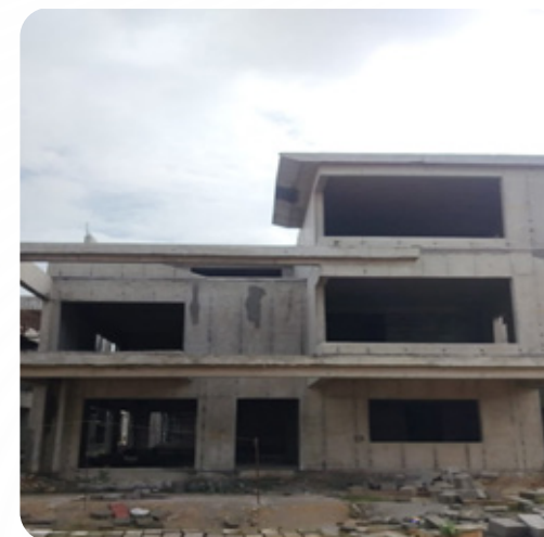
VILLA NO: 147 Brick Work Completed
