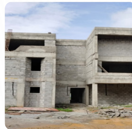
VILLA NO: 183 Brick Work Completed
