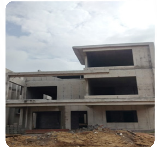
VILLA NO: 143 Block Work Completed
