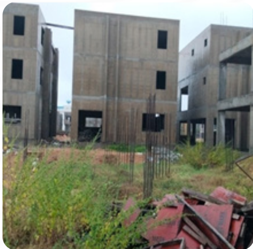
VILLA NO: 33 Plinth Beam Completed
