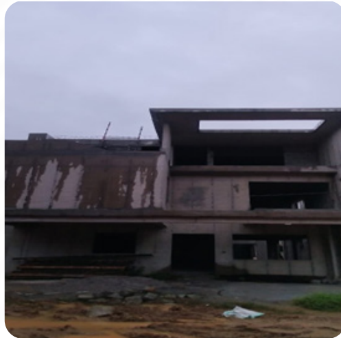
VILLA NO: 97 Block Work Completed
