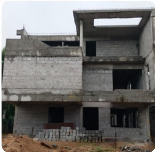
VILLA NO: 25 Brick Work Completed
