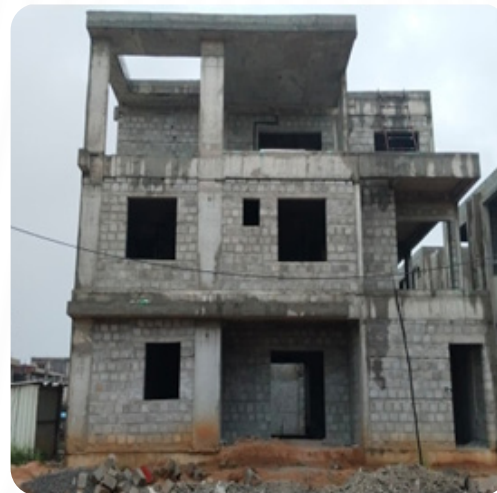
VILLA NO: 102 Brick Work Completed
