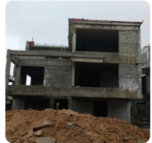
VILLA NO: 57 Brick Work Completed
