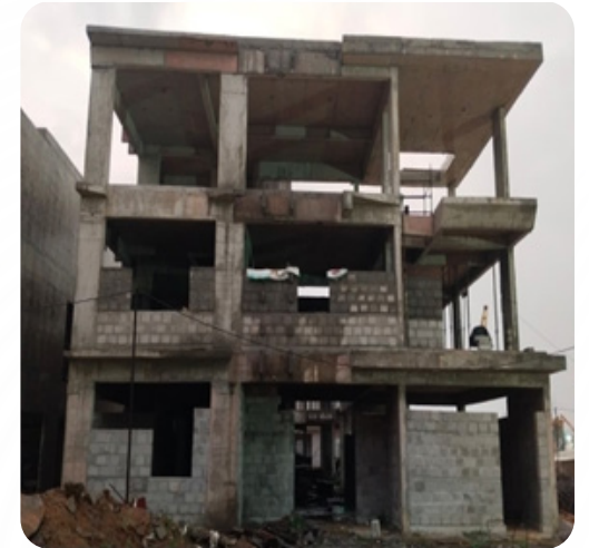
VILLA NO: 131 Slabs Completed
