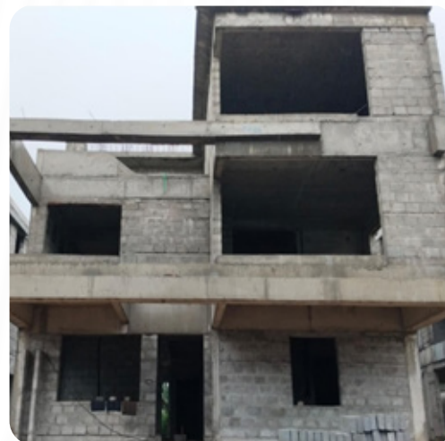
VILLA NO: 7 Brick Work Completed
