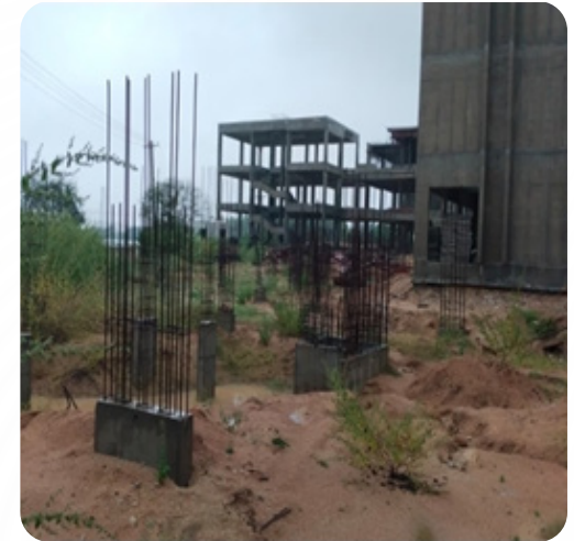
VILLA NO: 32 Plinth Beam Completed
