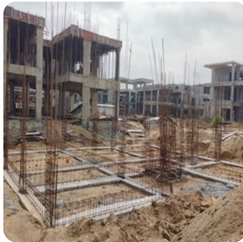
VILLA NO: 169 Plinth Work Completed
