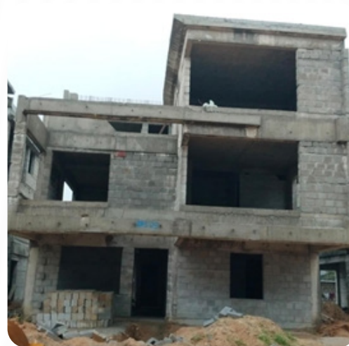
VILLA NO: 190 Brick Work Completed
