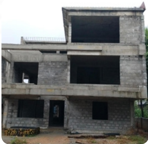
VILLA NO: 37 Brick Work Completed
