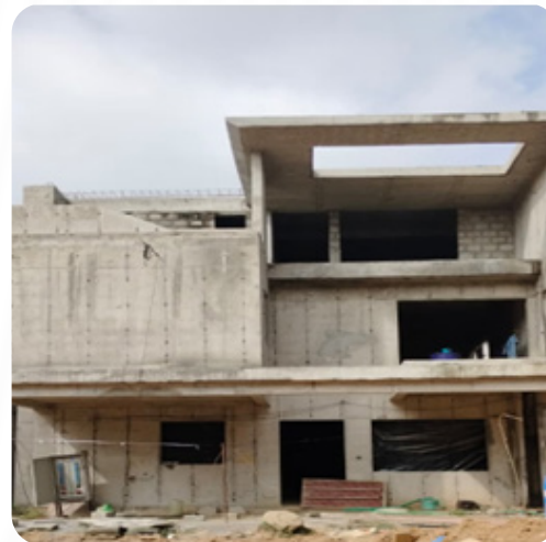
VILLA NO: 158 Block Work Completed
