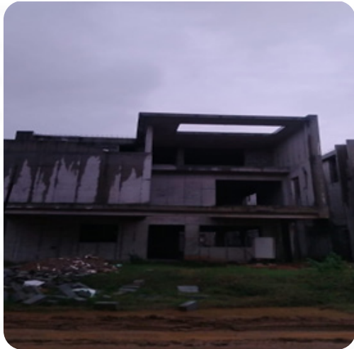
VILLA NO: 104 Block Work Completed
