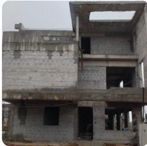
VILLA NO: 13 Brick Work Completed
