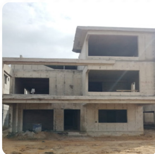
VILLA NO: 149 Block Work Completed
