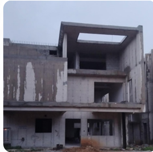
VILLA NO: 64 Block Work Completed
