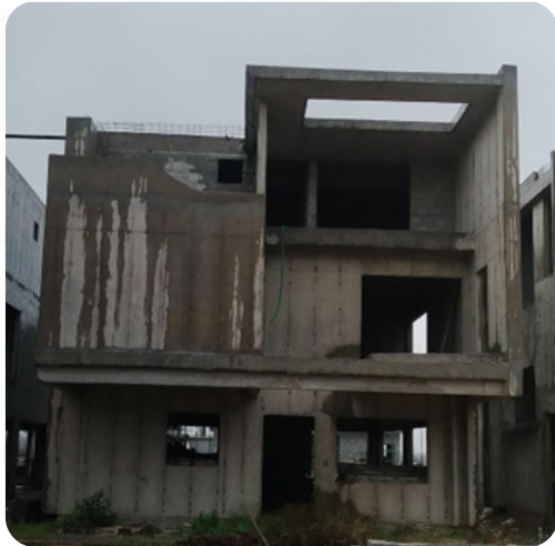
VILLA NO: 29 Block Work Completed
