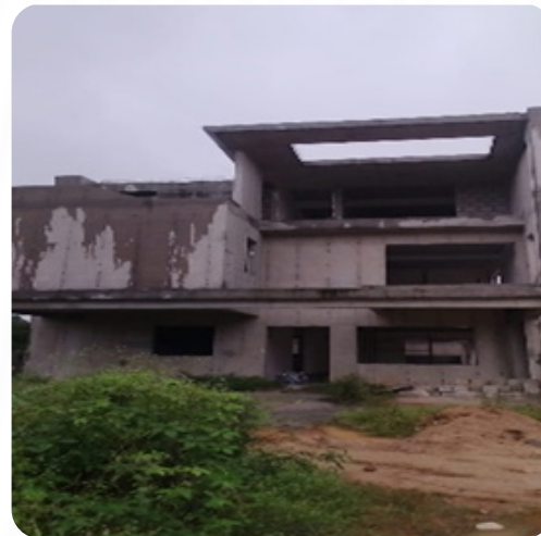
VILLA NO: 60 Block Work Completed
