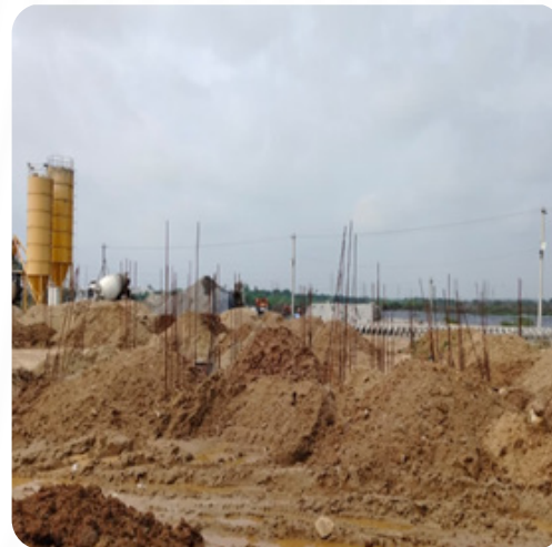
VILLA NO: 166 Plinth Work Completed
