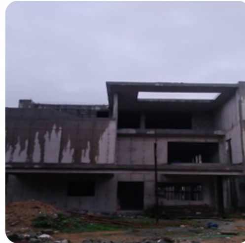
VILLA NO: 98 Block Work Completed
