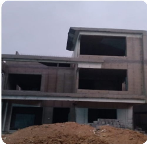
VILLA NO: 120 Block Work Completed
