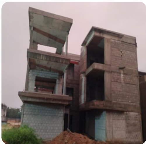
VILLA NO: 116 Brick Work Completed
