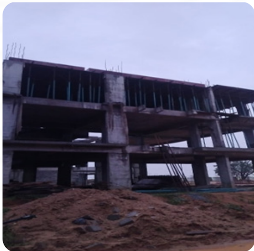
VILLA NO: 108 Slabs Work Completed
