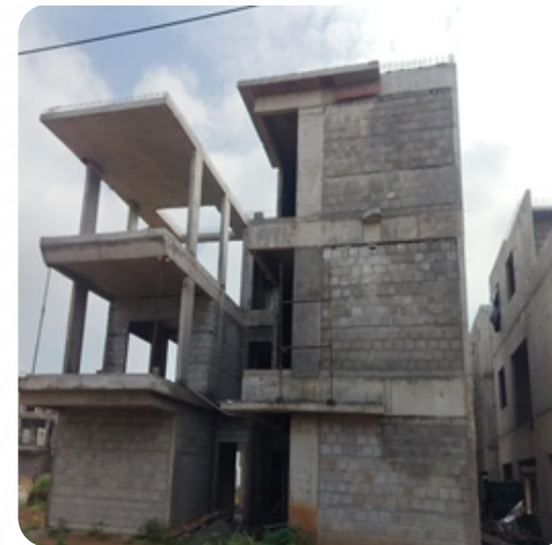
VILLA NO: 171 Plinth Work Completed
