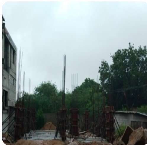
VILLA NO: 59 Plinth Work Completed
