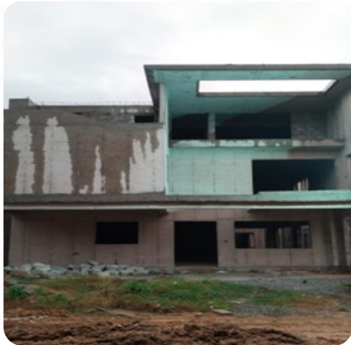
VILLA NO: 128 Block Work Completed
