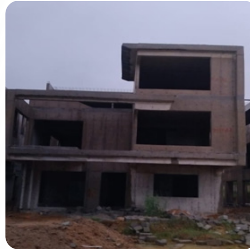
VILLA NO: 122 Block Work Completed
