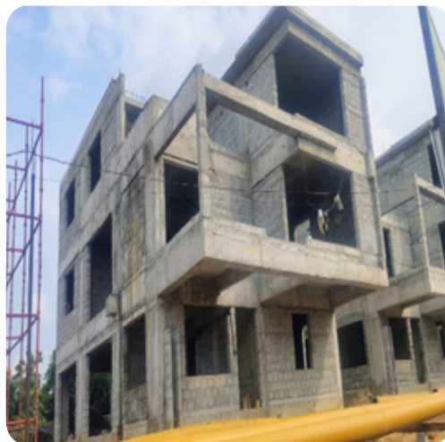
VILLA NO: 6 Brick Work Completed
