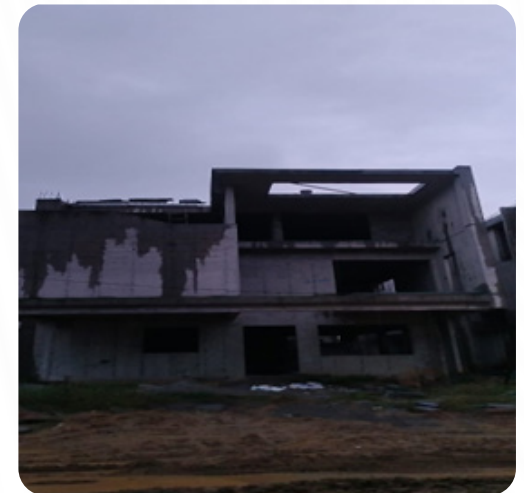
VILLA NO: 103 Block Work Completed
