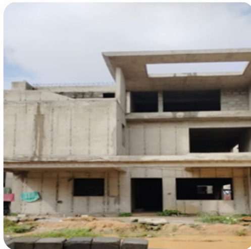
VILLA NO: 157 Block Work Completed
