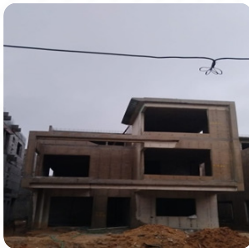
VILLA NO: 117 Block Work Completed
