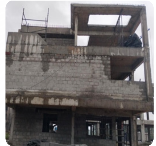
VILLA NO: 15 Brick Work Completed
