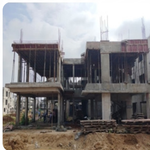
VILLA NO: 146 Slab Work Completed
