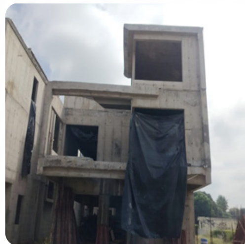
VILLA NO: 178 Block Work Completed
