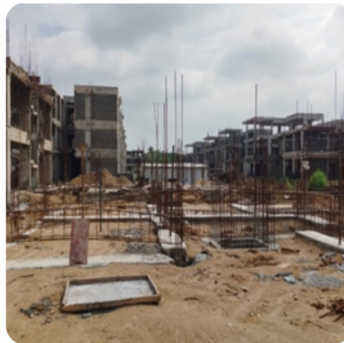
VILLA NO: 170 Plinth Work Completed
