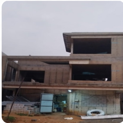
VILLA NO: 113 Block Work Completed
