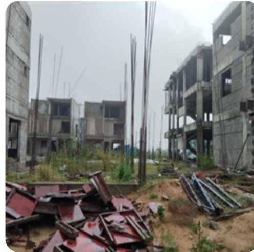
VILLA NO: 14 Plinth Beam Completed
