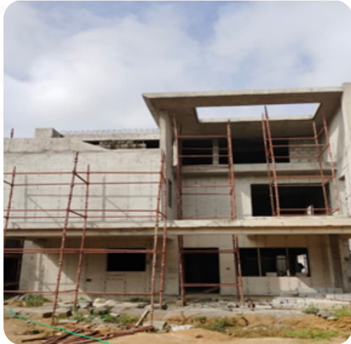
VILLA NO: 160 Block Work Completed
