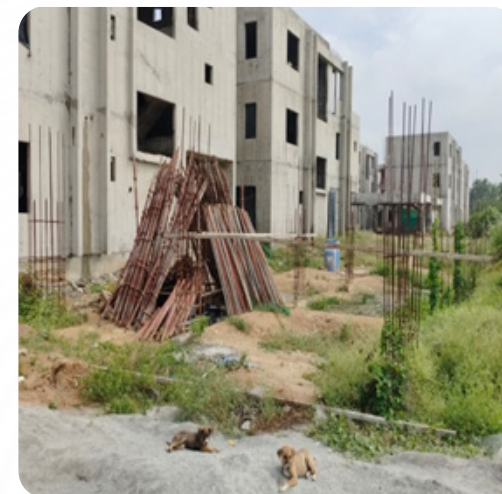
VILLA NO: 179 Plinth Work Completed
