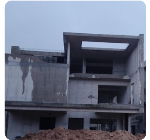
VILLA NO: 65 Block Work Completed
