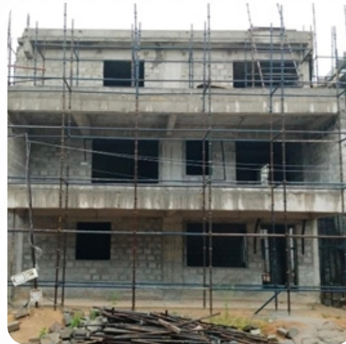
VILLA NO: 39 Brick Work Completed
