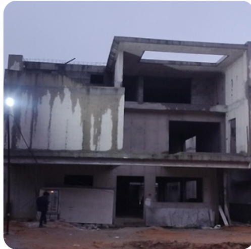
VILLA NO: 71 Block Work Completed
