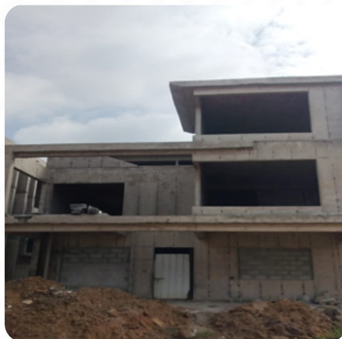
VILLA NO: 173 Block Work Completed
