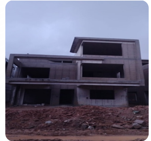
VILLA NO: 91 Block Work Completed
