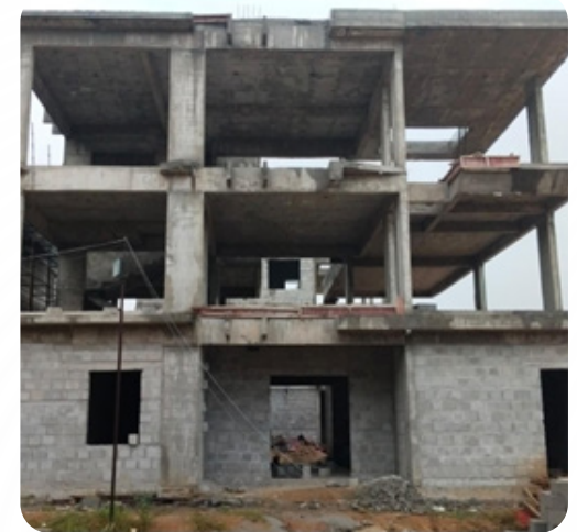
VILLA NO: 40 Slabs Completed
