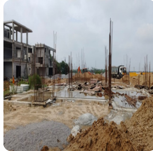
VILLA NO: 162 Plinth Work Completed
