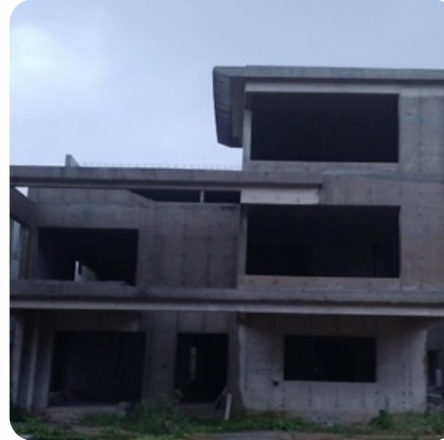
VILLA NO: 82 Block Work Completed
