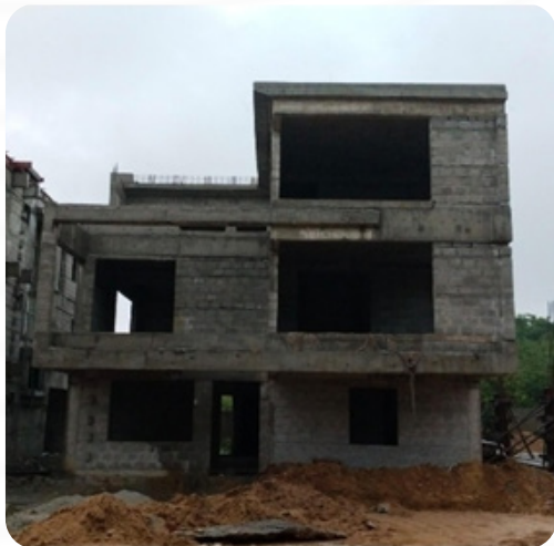
VILLA NO: 58 Brick Work Completed
