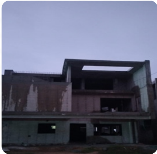
VILLA NO: 136 Block Work Completed
