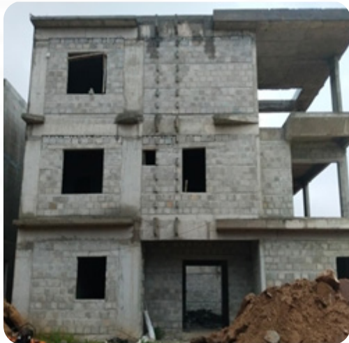
VILLA NO: 66 Brick Work Completed
