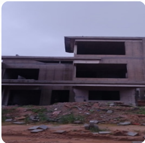
VILLA NO: 92 Block Work Completed
