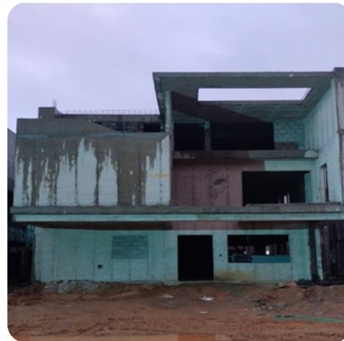
VILLA NO: 134 Block Work Completed
