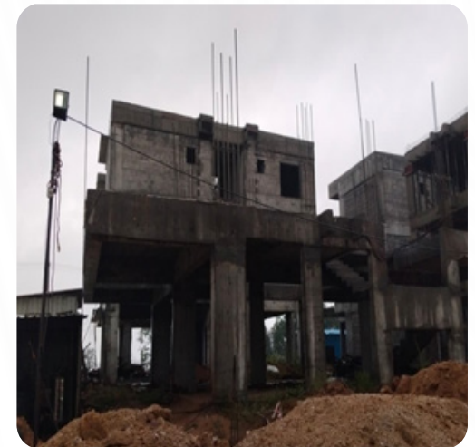
VILLA NO: 44 Slab Completed
