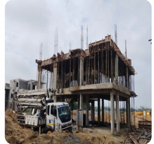
VILLA NO: 163 Slab Work Completed
