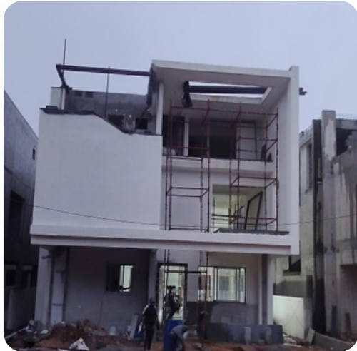
VILLA NO: 70 Block Work Completed
