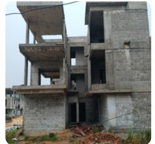
VILLA NO: 87 Brick Work Completed
