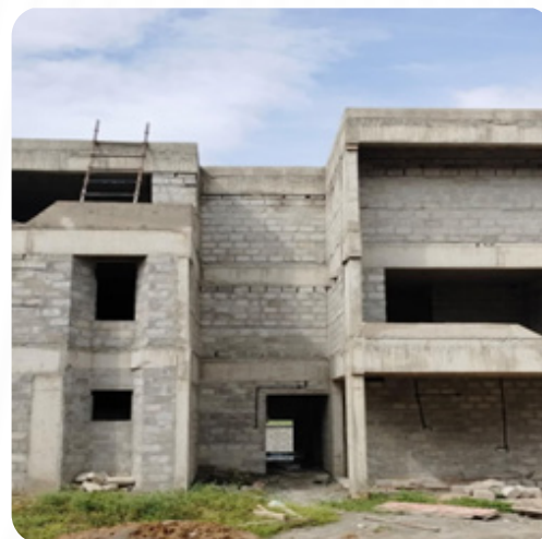
VILLA NO: 182 Brick Work Completed
