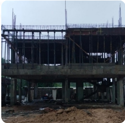
VILLA NO: 54 FF Slab Completed
