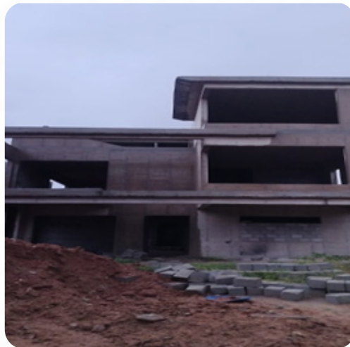
VILLA NO: 93 Block Work Completed
