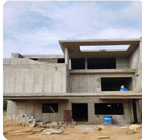
VILLA NO: 154 Block Work Completed
