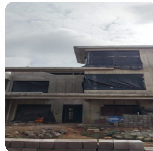
VILLA NO: 175 Block Work Completed
