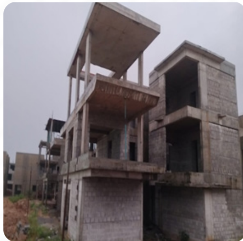
VILLA NO: 109 Brick Work Completed
