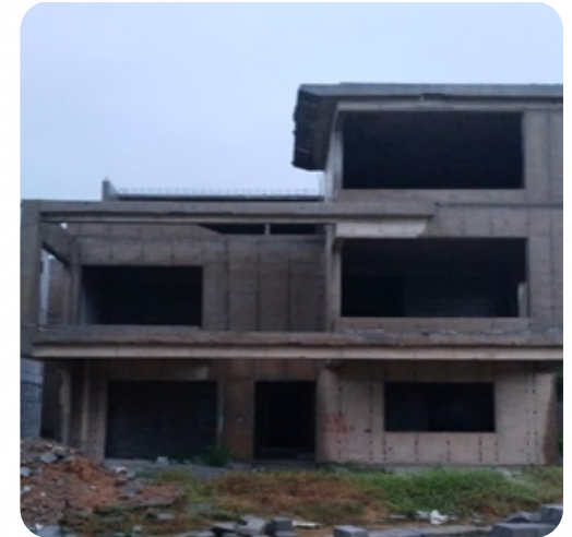
VILLA NO: 123 Block Work Completed
