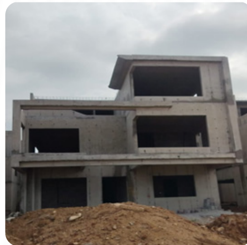
VILLA NO: 142 Block Work Completed
