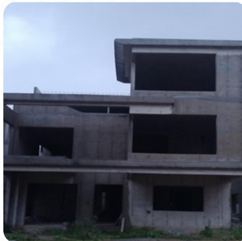
VILLA NO: 85 Block Work Completed
