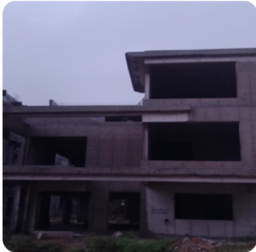
VILLA NO: 88 Block Work Completed
