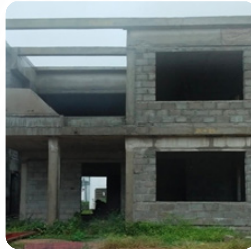
VILLA NO: 3 Brick Work Completed
