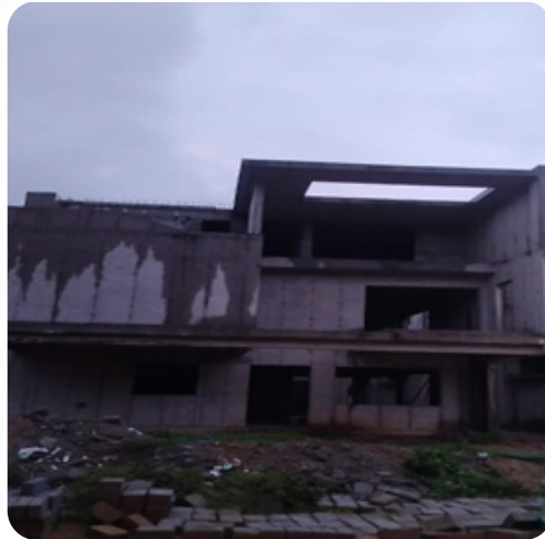
VILLA NO: 105 Block Work Completed
