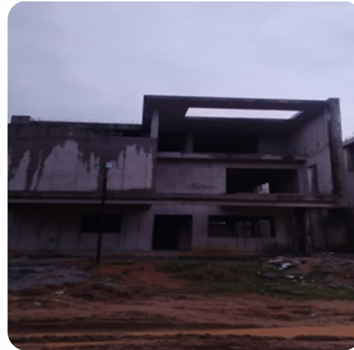
VILLA NO: 106 Block Work Completed
