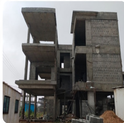
VILLA NO: 43 Slabs Completed & Brick Work in Process
