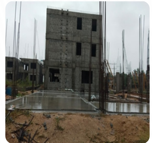
VILLA NO: 20 Grade Slab Completed
