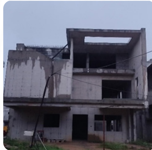
VILLA NO: 68 Block Work Completed
