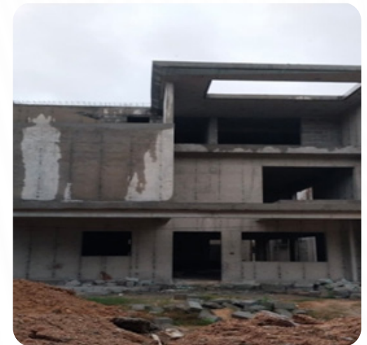
VILLA NO: 127 Block Work Completed
