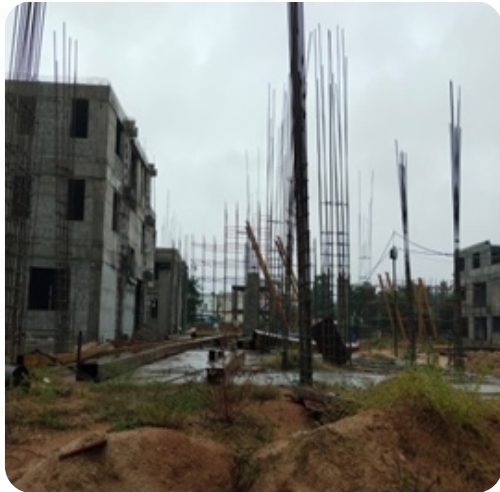
VILLA NO: 21 Grade Slab Completed
