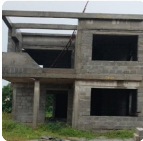
VILLA NO: 2 Brick Work Completed
