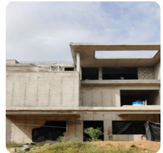
VILLA NO: 159 Block Work Completed
