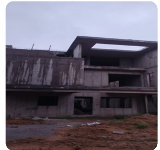
VILLA NO: 95 Block Work Completed
