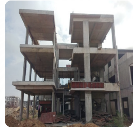
VILLA NO: 139 Slab Work Completed
