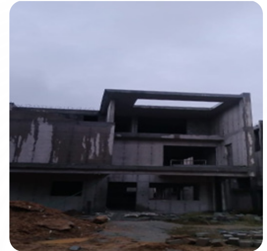
VILLA NO: 99 Block Work Completed
