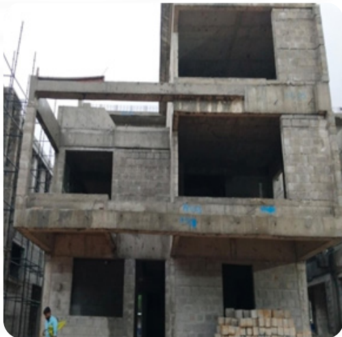
VILLA NO: 188 Brick Work Completed
