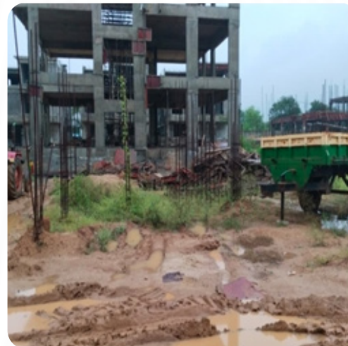
VILLA NO: 86 Plinth Work Completed
