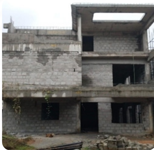
VILLA NO: 38 Brick Work Completed
