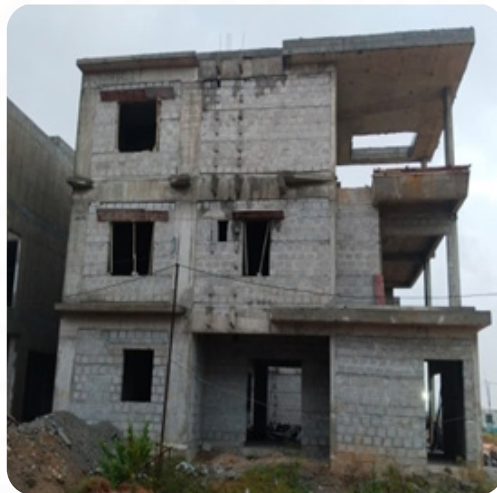
VILLA NO: 101 Brick Work Completed
