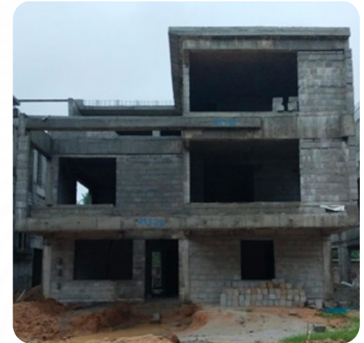
VILLA NO: 48 Brick Work Completed
