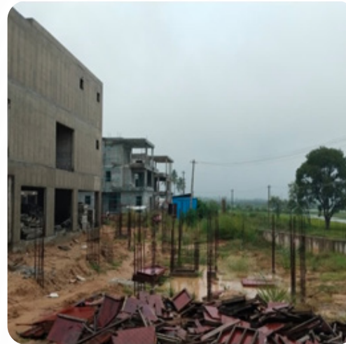
VILLA NO: 31 Plinth Beam Completed
