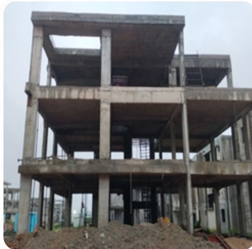
VILLA NO: 67 Slabs Completed
