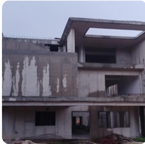
VILLA NO: 63 Block Work Completed
