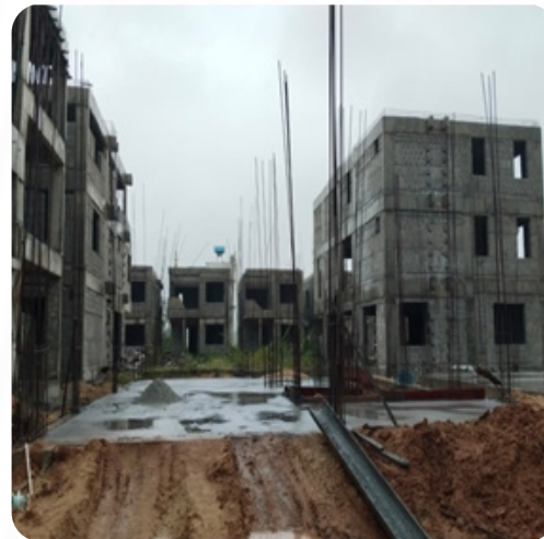
VILLA NO: 19 Grade Slab Completed
