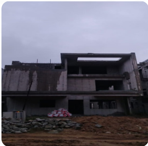
VILLA NO: 100 Block Work Completed
