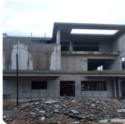
VILLA NO: 130 Block Work Completed
