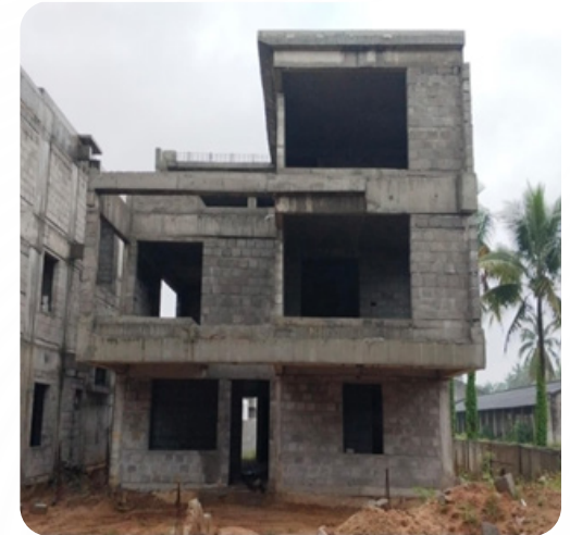
VILLA NO: 24 Brick Work Completed
