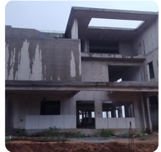
VILLA NO: 73 Block Work Completed
