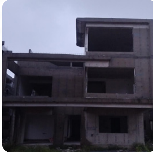
VILLA NO: 81 Block Work Completed
