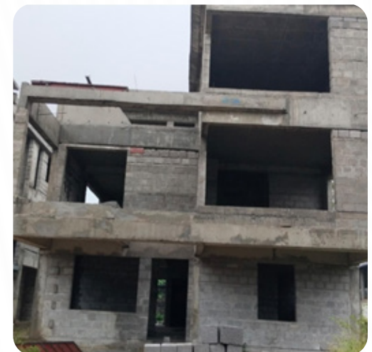
VILLA NO: 8 Brick Work Completed
