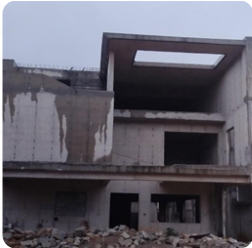
VILLA NO: 62 Block Work Completed
