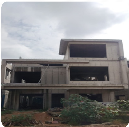
VILLA NO: 176 Block Work Completed
