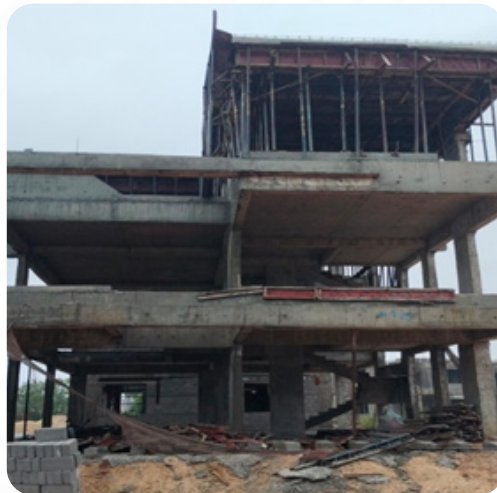
VILLA NO: 18 Slabs Completed
