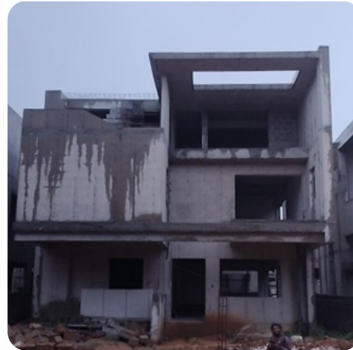
VILLA NO: 72 Block Work Completed
