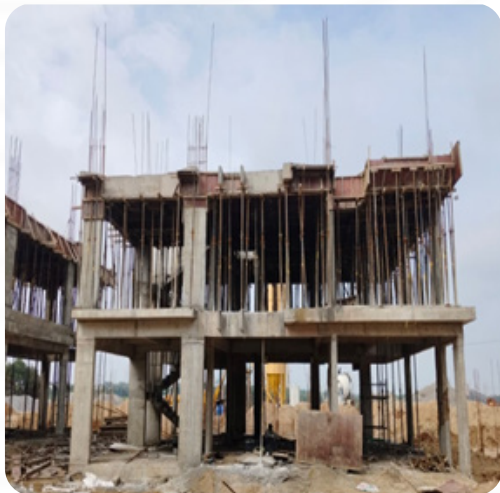
VILLA NO: 164 Slab Work Completed
