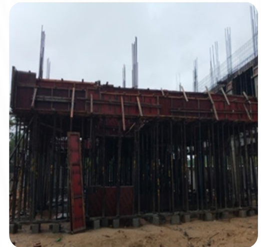
VILLA NO: 53 FF Slab Completed
