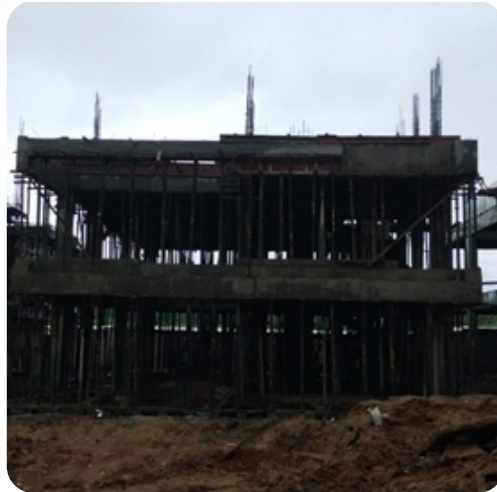
VILLA NO: 55 FF Slab Completed
