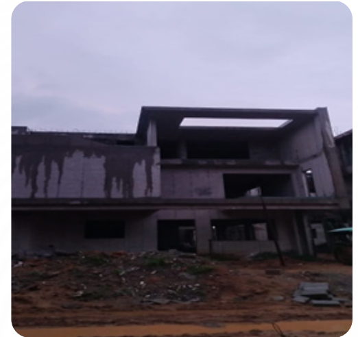
VILLA NO: 107 Block Work Completed
