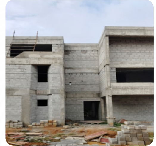
VILLA NO: 187 Brick Work Completed
