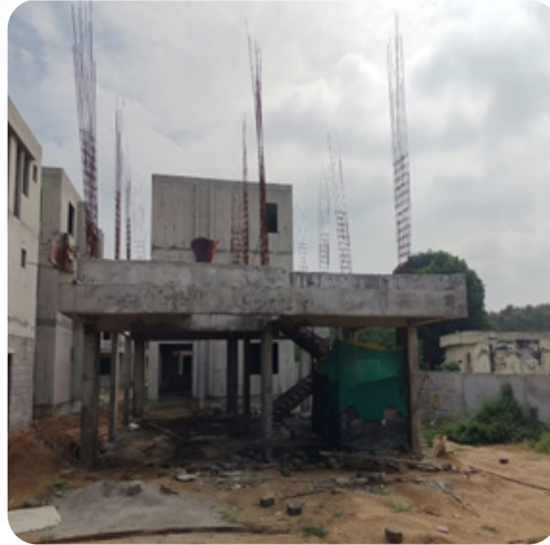
VILLA NO: 153 Plinth Work Completed
