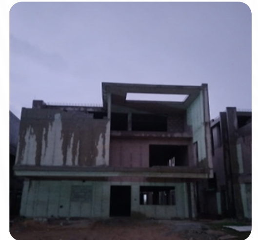
VILLA NO: 135 Block Work Completed
