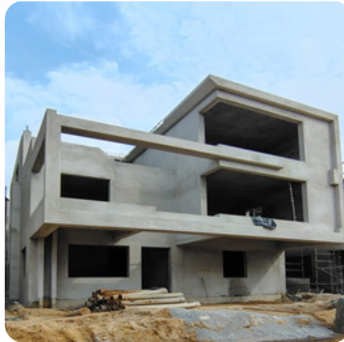
VILLA NO: 46 Brick Work Completed
