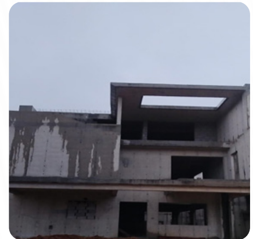
VILLA NO: 61 Block Work Completed
