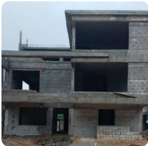
VILLA NO: 49 Brick Work Completed
