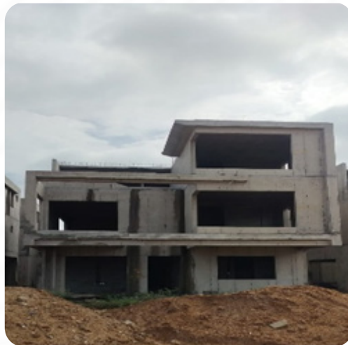
VILLA NO: 141 Block Work Completed
