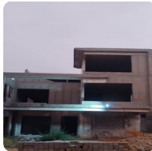
VILLA NO: 114 Block Work Completed
