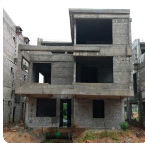
VILLA NO: 23 Brick Work Completed
