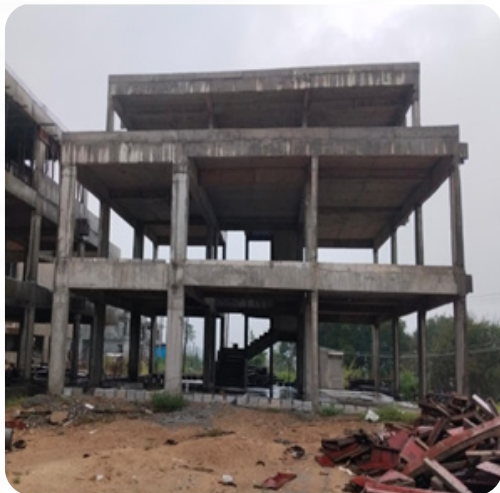
VILLA NO: 17 Slabs Completed
