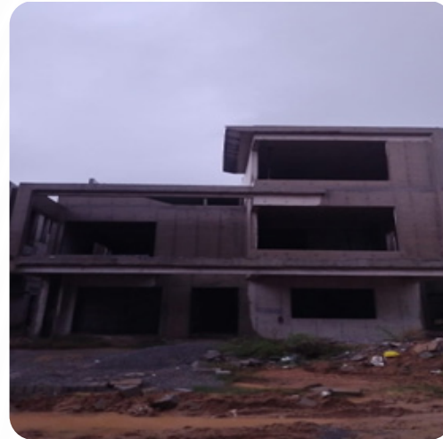
VILLA NO: 90 Block Work Completed
