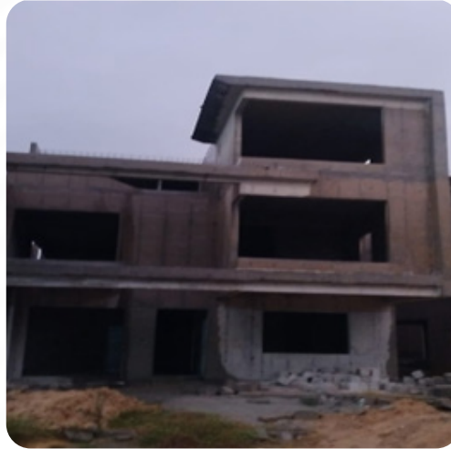
VILLA NO: 121 Block Work Completed
