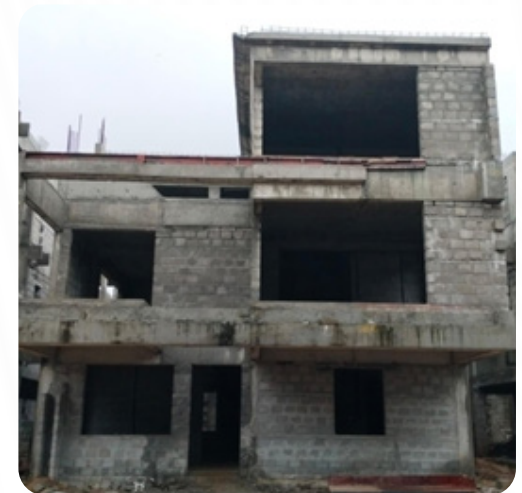
VILLA NO: 36 Brick Work Completed
