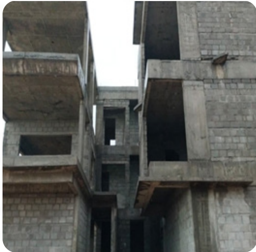
VILLA NO: 45 Brick Work Completed
