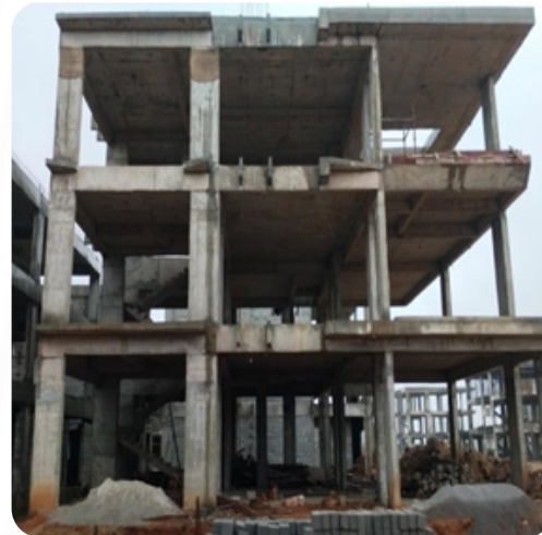
VILLA NO: 27 Slab Work Completed
