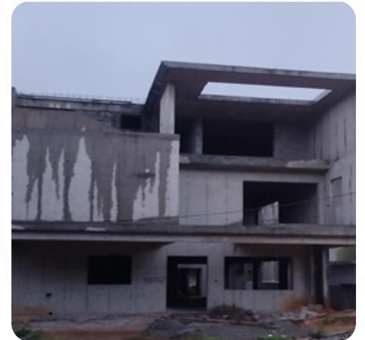
VILLA NO: 69 Block Work Completed
