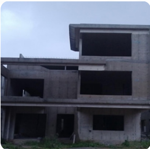
VILLA NO: 84 Block Work Completed
