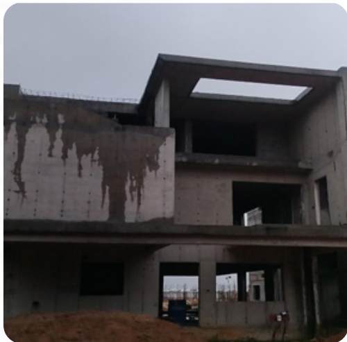
VILLA NO: 74 Block Work Completed
