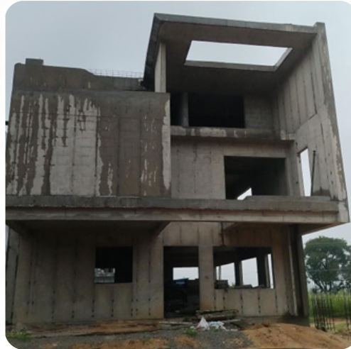
VILLA NO: 30 Block Work Completed
