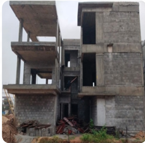
VILLA NO: 22 Brick Work Completed
