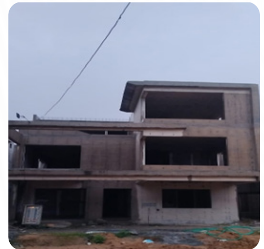
VILLA NO: 111 Block Work Completed
