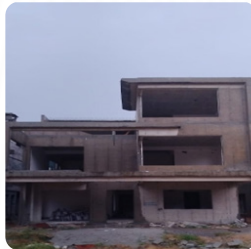
VILLA NO: 110 Block Work Completed
