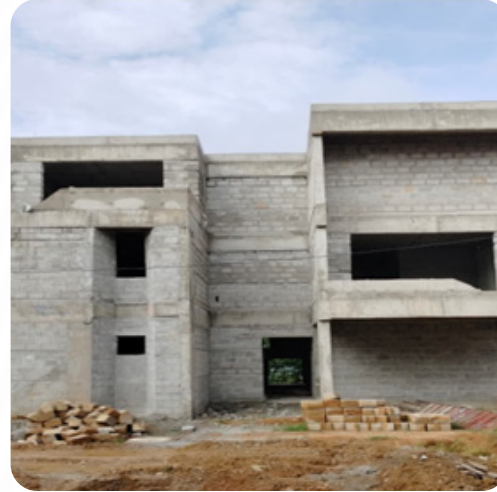
VILLA NO: 186 Brick Work Completed
