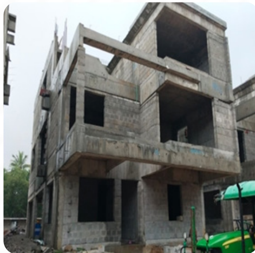
VILLA NO: 189 Brick Work Completed
