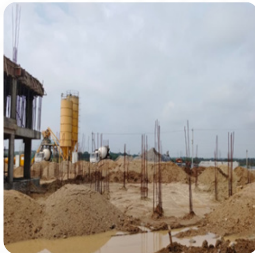
VILLA NO: 165 Plinth Work Completed
