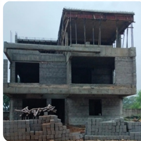
VILLA NO: 51 Slab Work Completed
