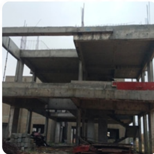
VILLA NO: 34 Slabs Completed
