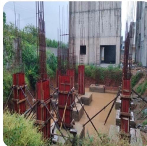
VILLA NO: 94 Footing Completed
