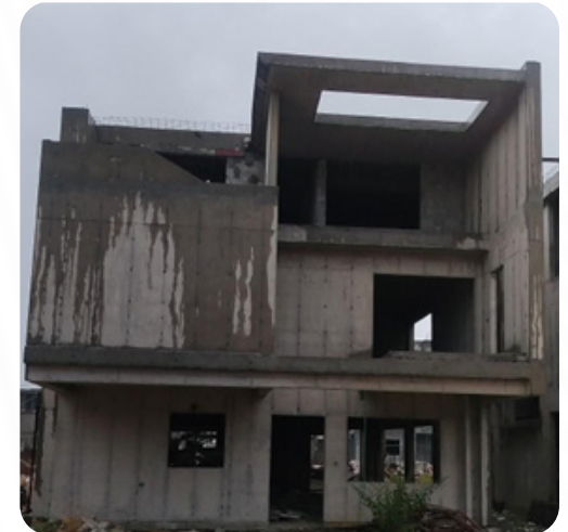
VILLA NO: 28 Block Work Completed
