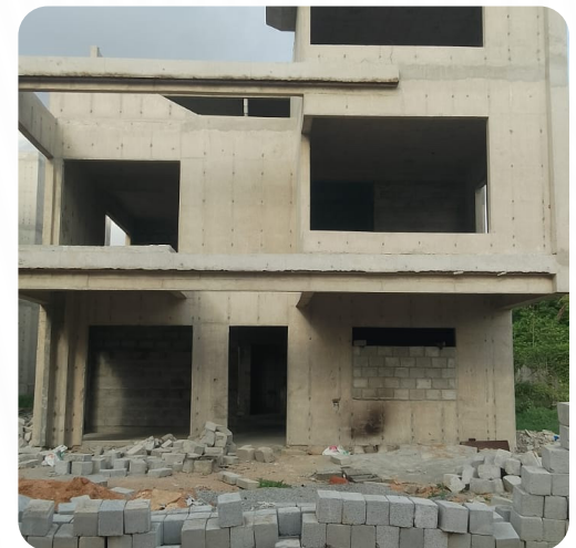
VILLA NO: 94 (Footings Completed)
