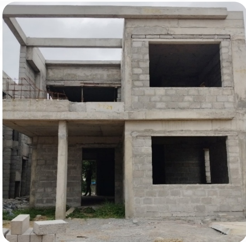
VILLA NO: 5 (Structure Completed)
