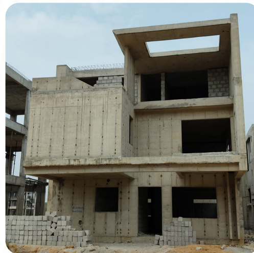
VILLA NO: 133 (Structure Completed)
