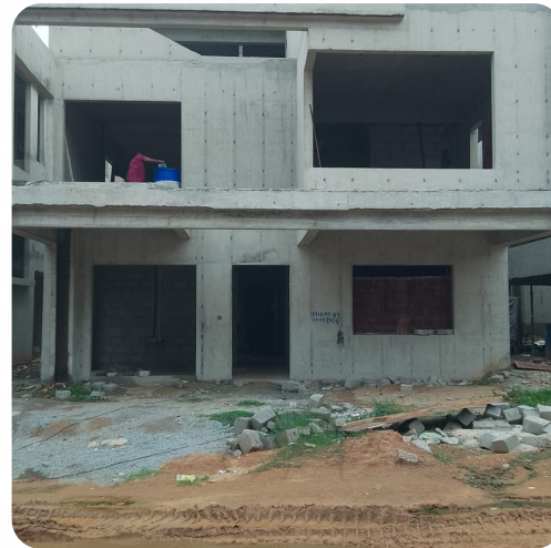
VILLA NO: 89 (Structure Completed)
