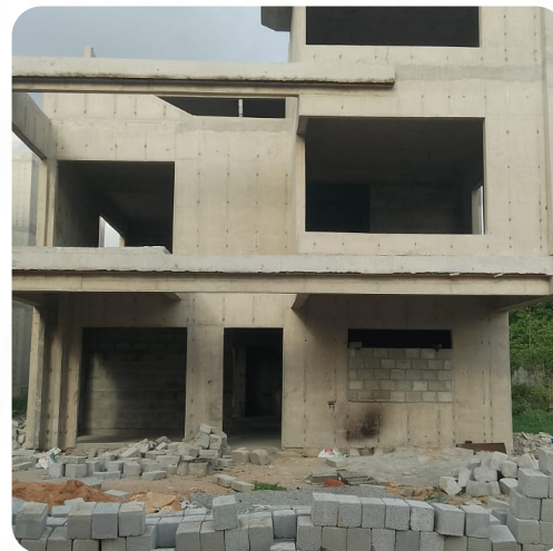
VILLA NO: 93 (Structure Completed)
