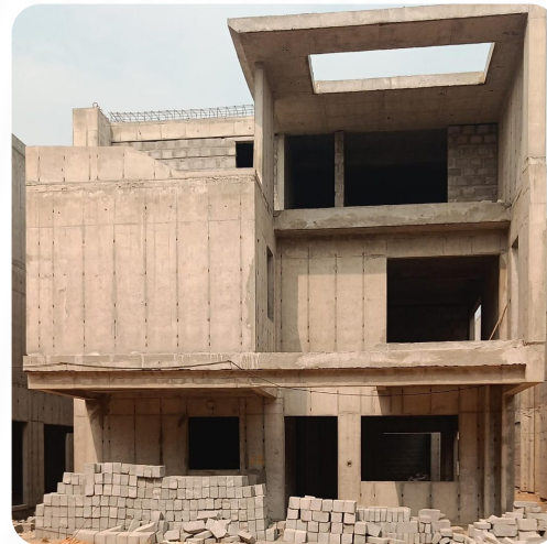
VILLA NO: 157 (Structure Completed)
