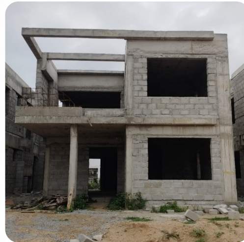
VILLA NO: 3 (Structure Completed)
