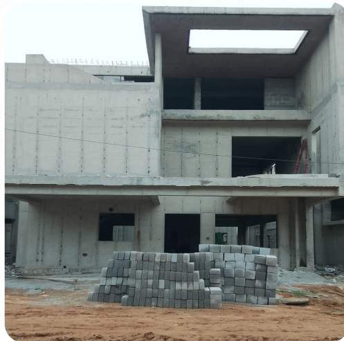
VILLA NO: 96 (Structure Completed)
