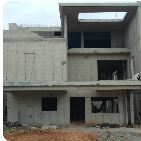
VILLA NO: 64 (Structure Completed)
