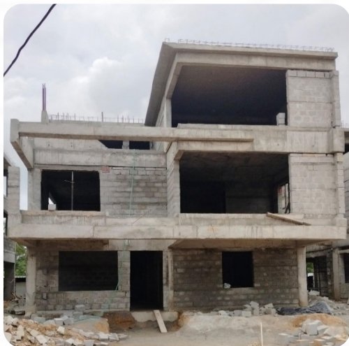
VILLA NO: 49 (Structure Completed)
