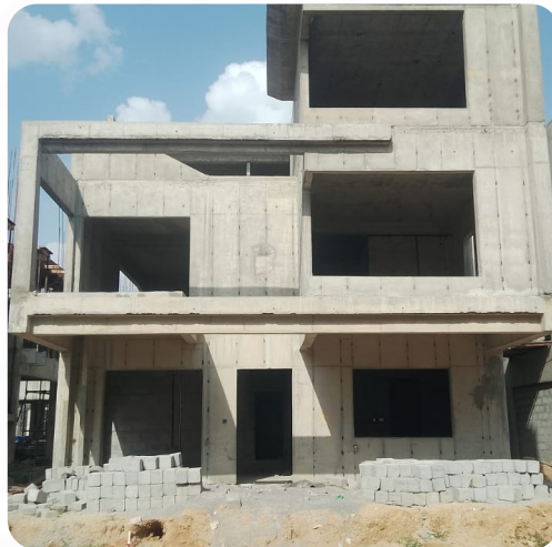
VILLA NO: 172 (Structure Completed)
