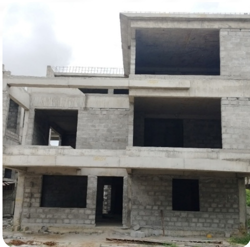
VILLA NO: 37 (Structure Completed)
