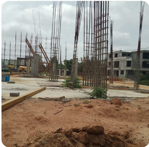
VILLA NO: 21 (Grade Slab Completed)
