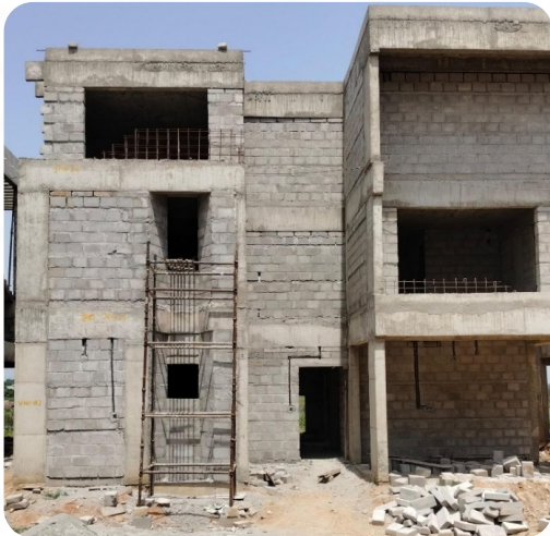
VILLA NO: 183 (Structure Completed)
