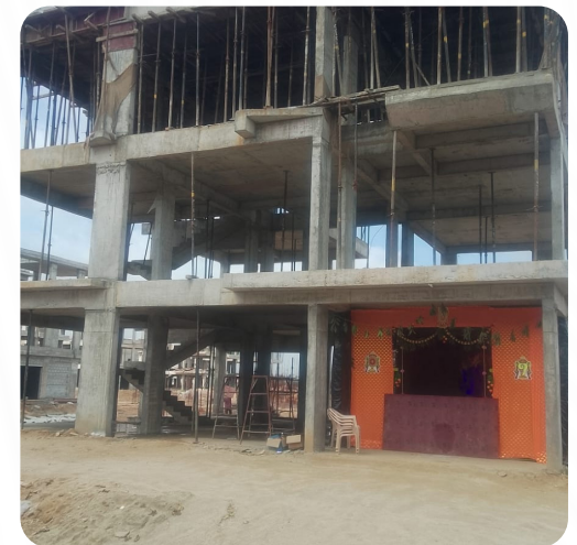
VILLA NO: 77 (SF Slab Completed)
