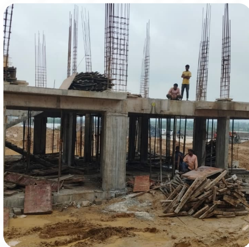
VILLA NO: 164 (GF Slab Completed)
