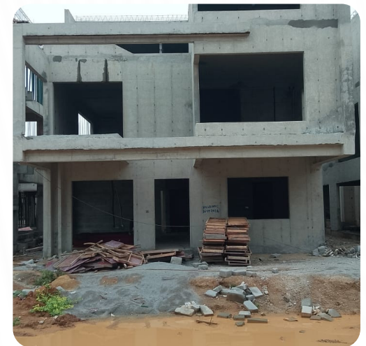
VILLA NO: 110 (Structure Completed)
