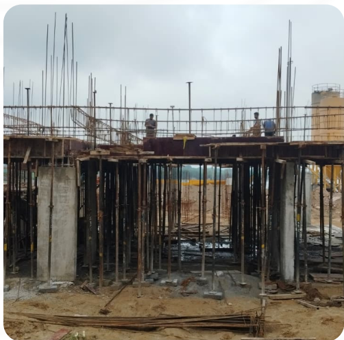
VILLA NO: 163 (GF Columns Completed)
