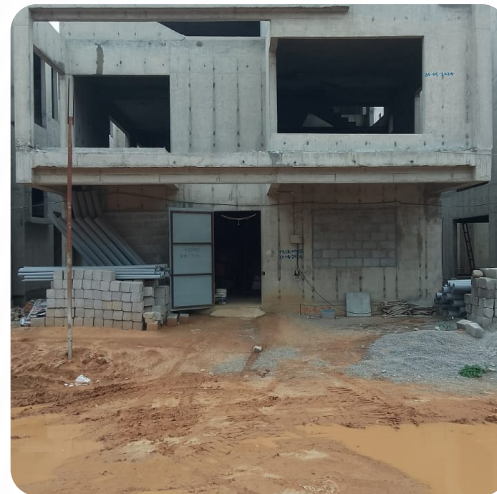
VILLA NO: 113 (Structure Completed)
