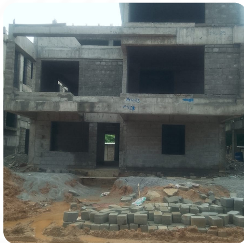
VILLA NO: 188 (SF Slab Completed)
