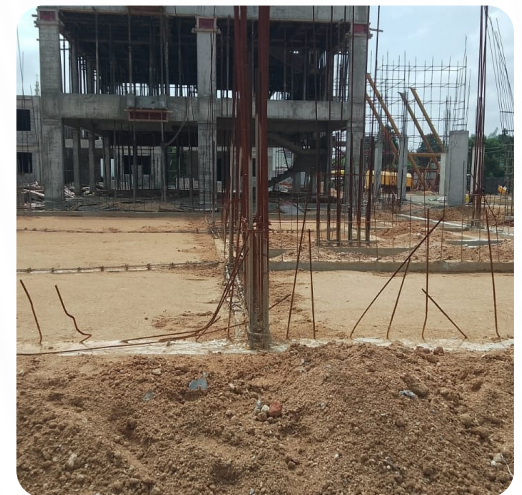
VILLA NO: 20 (Plinth Beam Completed)
