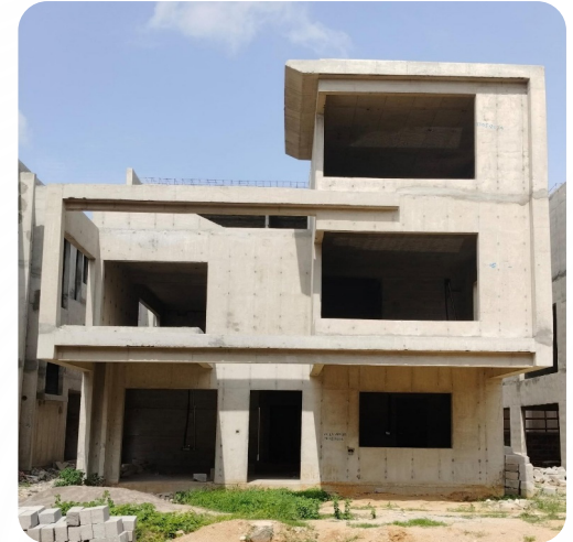
VILLA NO: 82 (Structure Completed)
