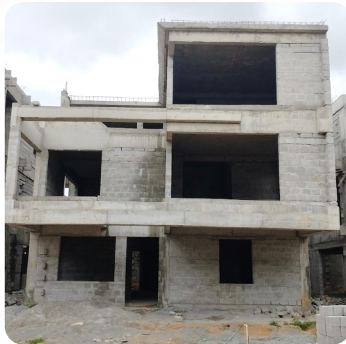
VILLA NO: 46 (Structure Completed)
