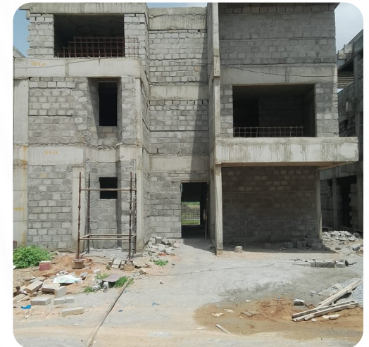
VILLA NO: 182 (Structure Completed)
