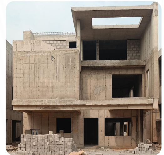
VILLA NO: 158 (Structure Completed)
