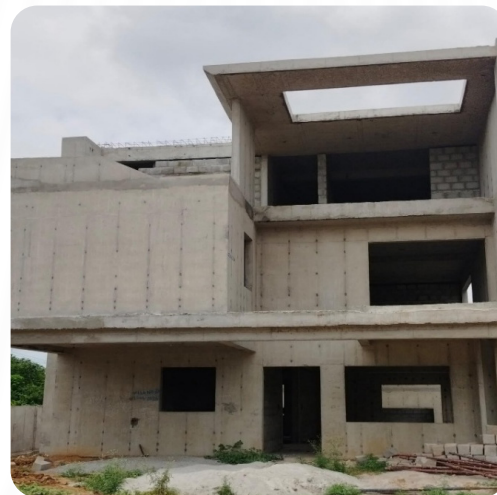
VILLA NO: 60 (Structure Completed)
