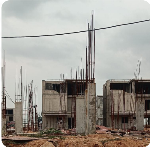
VILLA NO: 12 (Ground Floor Columns Completed)
