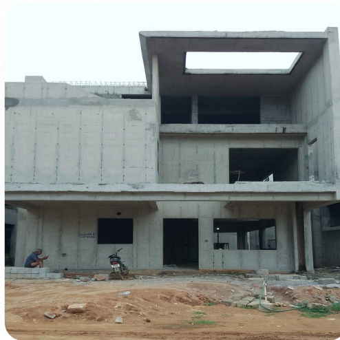
VILLA NO: 71 (Structure Completed)
