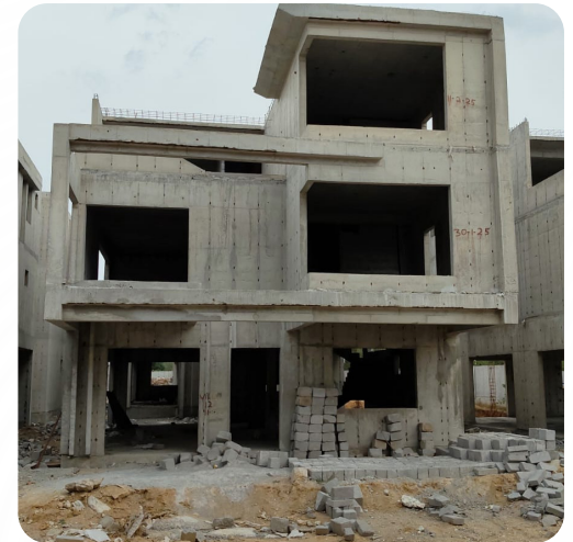
VILLA NO: 122 (Structure Completed)
