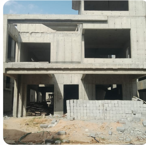
VILLA NO: 177 (Structure Completed)
