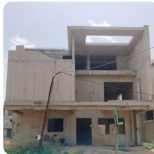
VILLA NO: 68 (Structure Completed)
