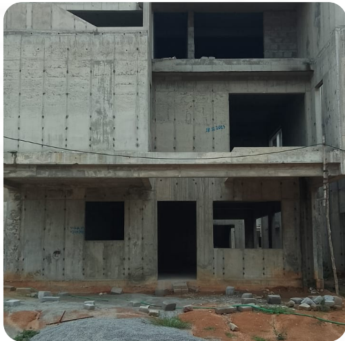
VILLA NO: 103 (Structure Completed)
