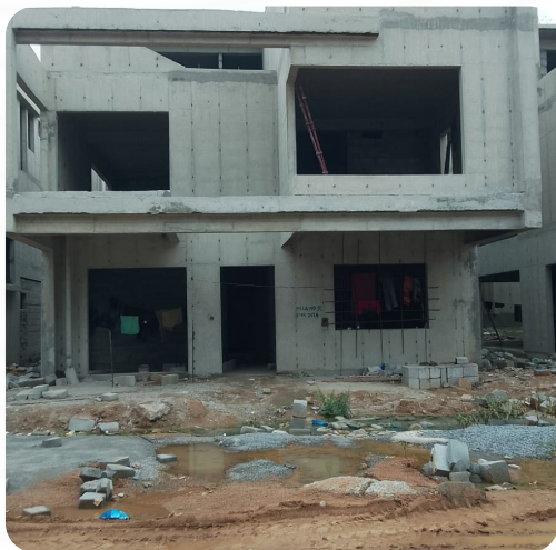
VILLA NO: 91 (Structure Completed)
