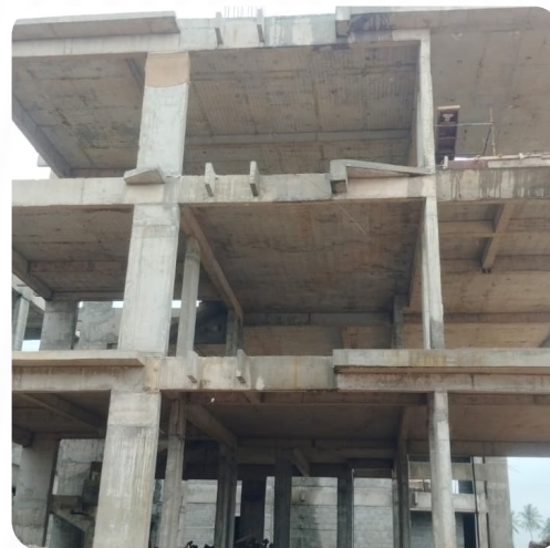
VILLA NO: 27 (Structure Completed)
