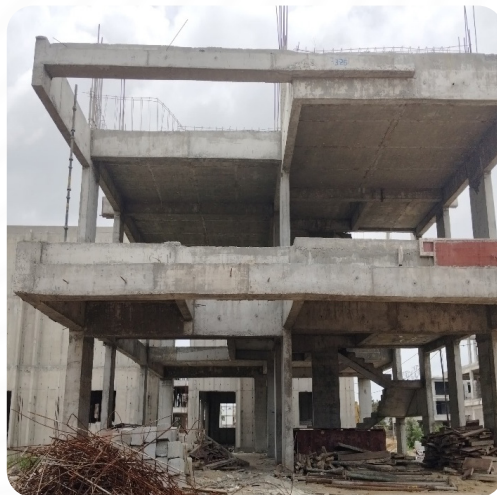
VILLA NO: 34 (FF slab Completed)
