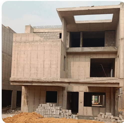
VILLA NO: 156 (Structure Completed)
