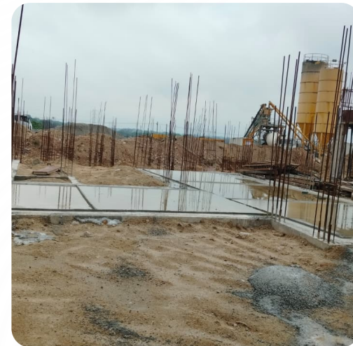
VILLA NO: 162 (Grade Slab Completed)
