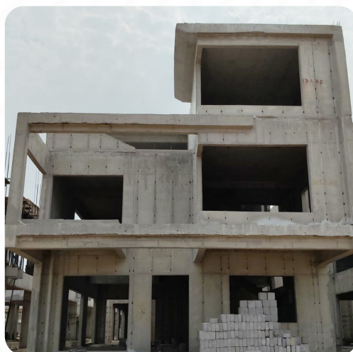
VILLA NO: 140 (Structure Completed)
