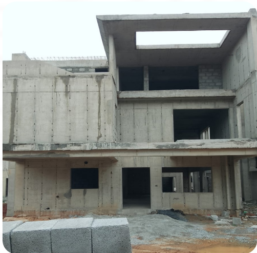
VILLA NO: 95 (Structure Completed)
