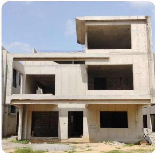
VILLA NO: 83 (Structure Completed)
