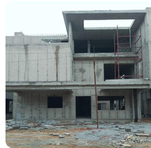
VILLA NO: 98 (Structure Completed)
