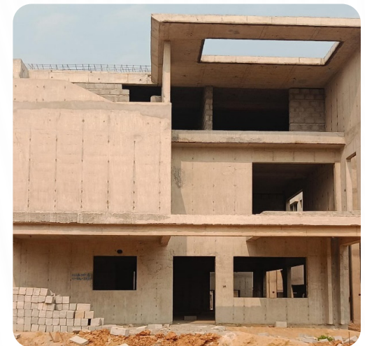
VILLA NO: 61 (Structure Completed)
