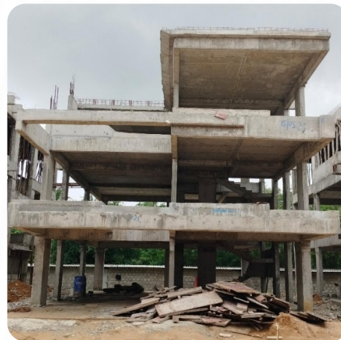
VILLA NO: 189 (SF Slab Completed)
