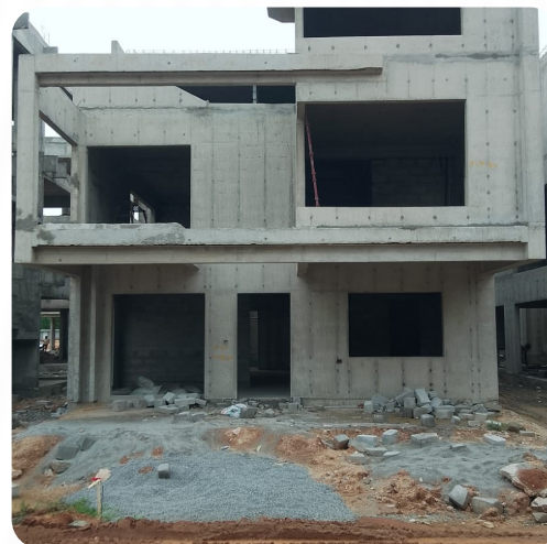
VILLA NO: 117 (Structure Completed)
