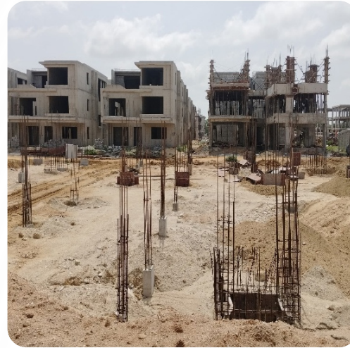
VILLA NO: 169 (Pedestals Completed)
