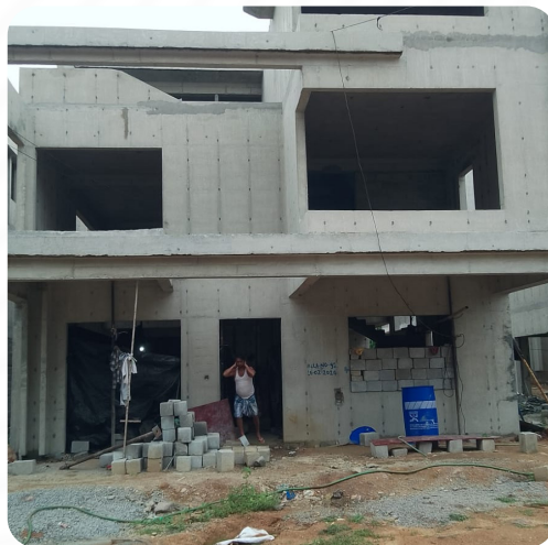
VILLA NO: 92 (Structure Completed)
