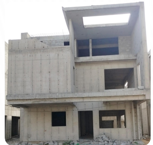
VILLA NO: 126 (Structure Completed)
