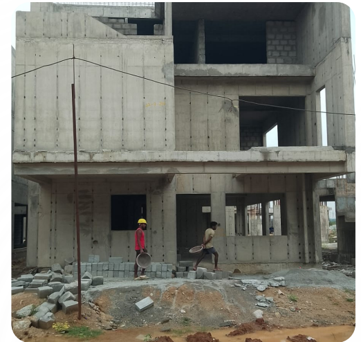
VILLA NO: 130 (Structure Completed)
