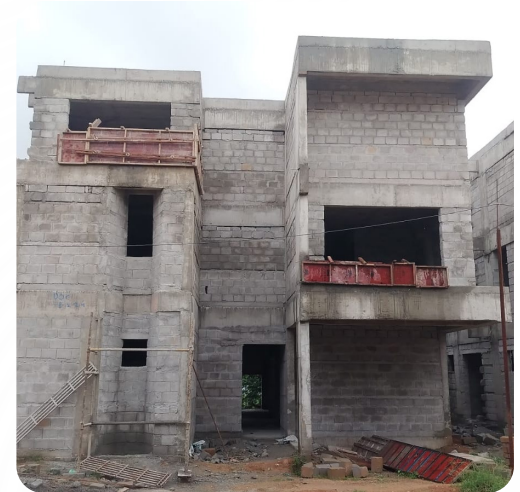
VILLA NO: 186 (Structure Completed)
