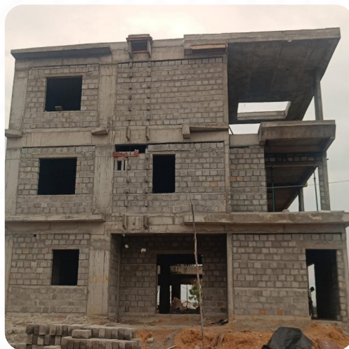
VILLA NO: 42 (Structure Completed)
