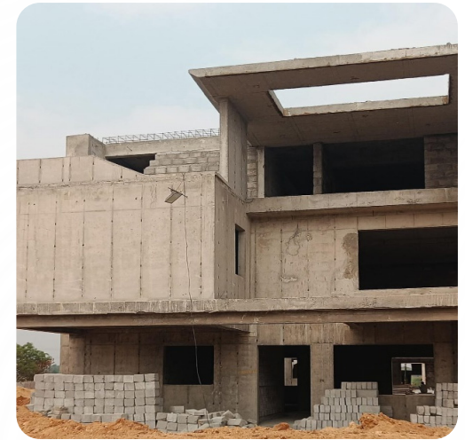
VILLA NO: 154 (Structure Completed)
