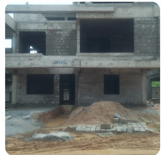
VILLA NO: 190 (SF Slab Completed)
