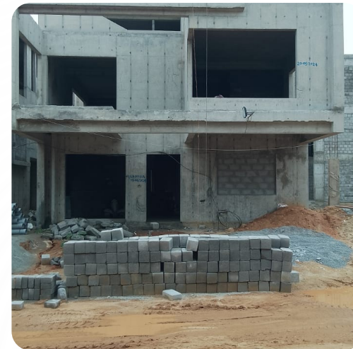
VILLA NO: 114 (Structure Completed)
