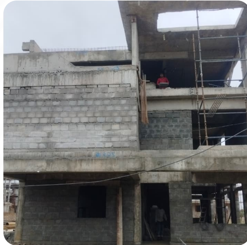
VILLA NO: 13 (Structure Completed)
