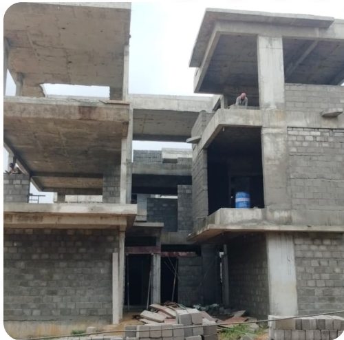
VILLA NO: 87 (Structure Completed)
