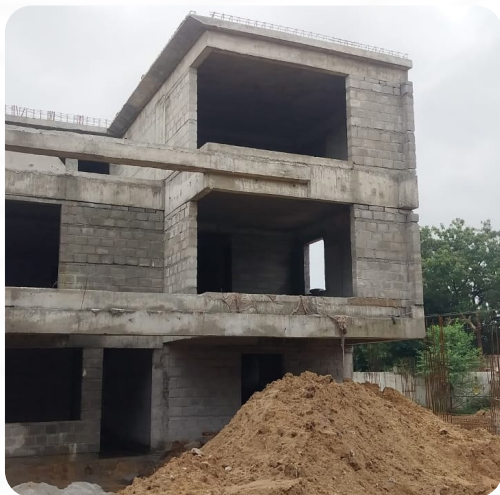
VILLA NO: 58 (Structure Completed)
