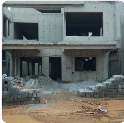
VILLA NO: 112 (Structure Completed)
