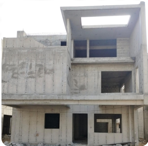
VILLA NO: 127 (Structure Completed)
