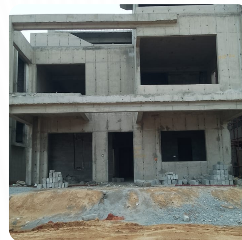
VILLA NO: 142 (Structure Completed)
