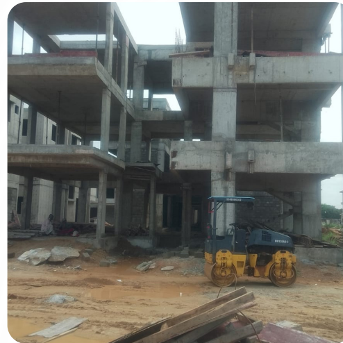
VILLA NO: 145 (SF Slab Completed)
