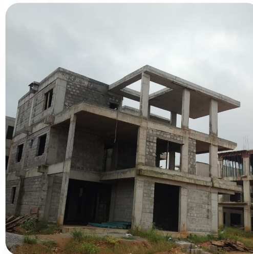
VILLA NO: 109 (Structure Completed)
