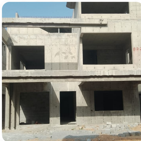
VILLA NO: 148 (Structure Completed)
