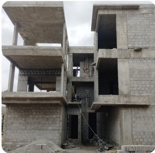
VILLA NO: 45 (Structure Completed)
