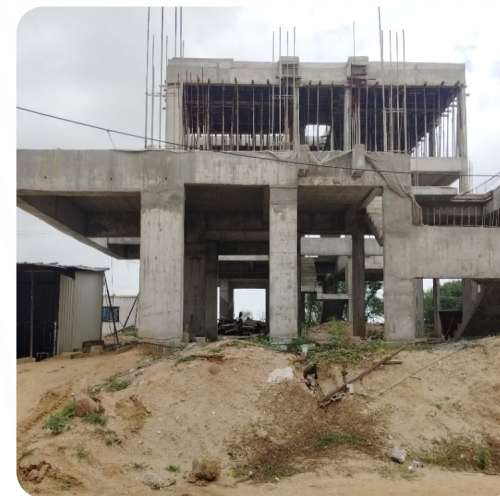
VILLA NO: 44 (GF Slab Completed)
