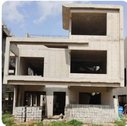
VILLA NO: 88 (Structure Completed)
