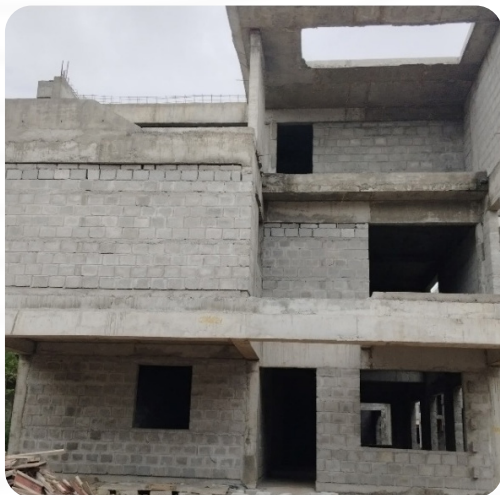
VILLA NO: 25 (Structure Completed)
