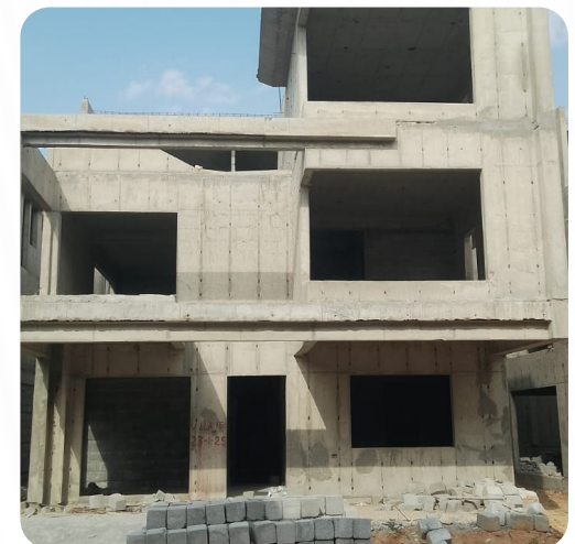
VILLA NO: 150 (Structure Completed)
