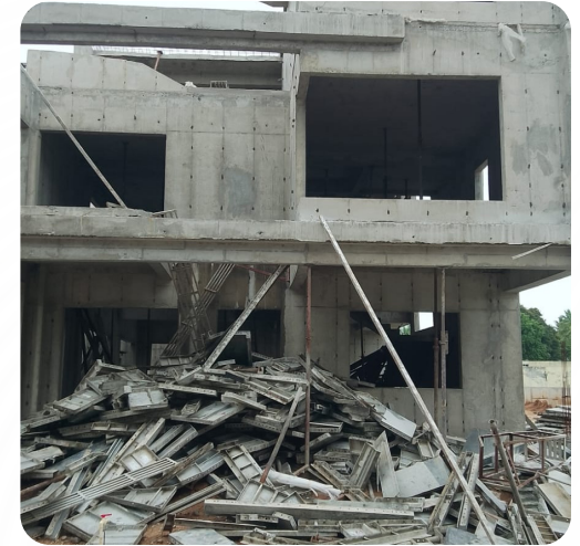
VILLA NO: 178 (Structure Completed)
