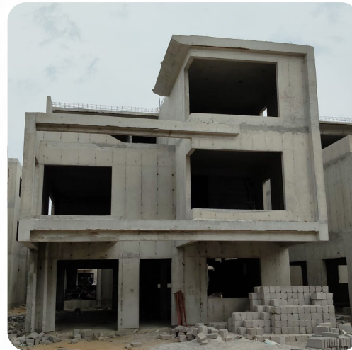
VILLA NO: 121 (Structure Completed)
