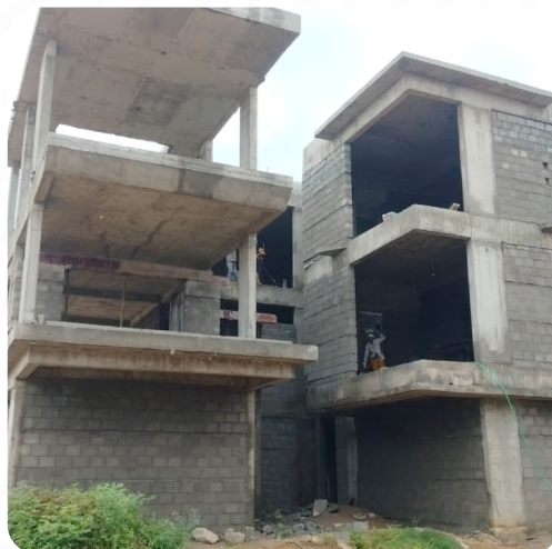
VILLA NO: 116 (Structure Completed)
