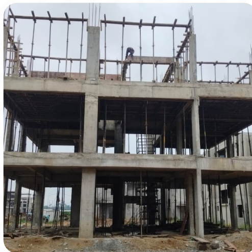
VILLA NO: 75 (Structure Completed)
