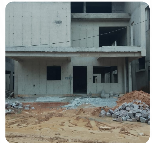
VILLA NO: 69 (Structure Completed)
