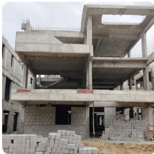
VILLA NO: 26 (Structure Completed)
