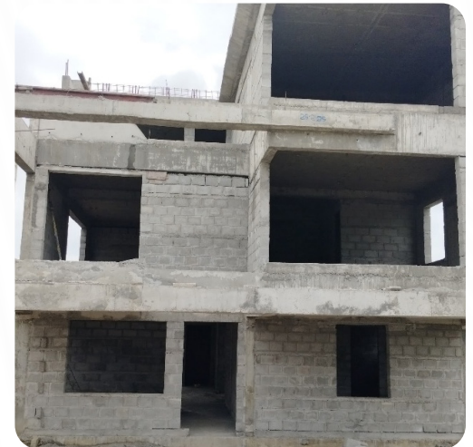
VILLA NO: 8 (Structure Completed)
