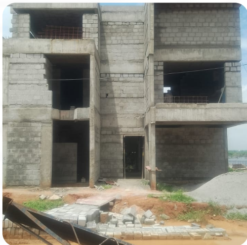
VILLA NO: 187 (Structure Completed)
