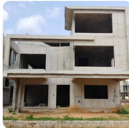
VILLA NO: 85 (Structure Completed)
