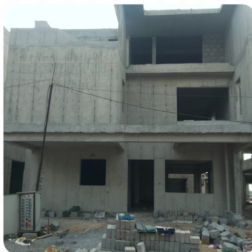
VILLA NO: 100 (Structure Completed)
