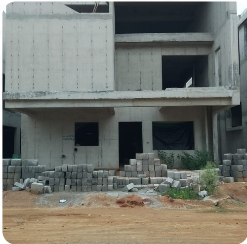
VILLA NO: 62 (Structure Completed)
