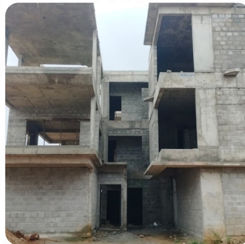
VILLA NO: 35 (Structure Completed)
