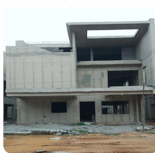
VILLA NO: 97 (Structure Completed)
