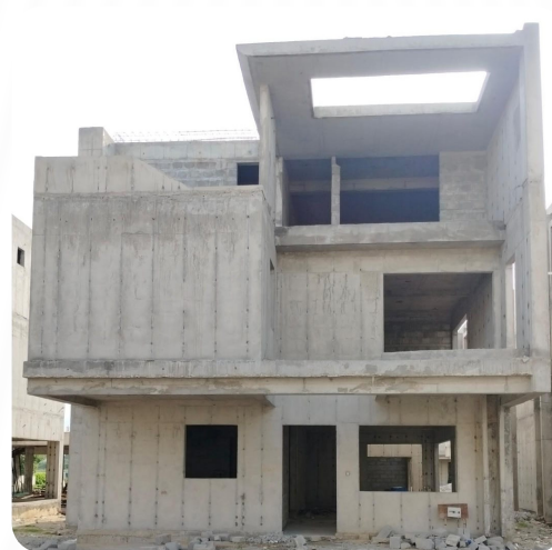
VILLA NO: 125 (Structure Completed)
