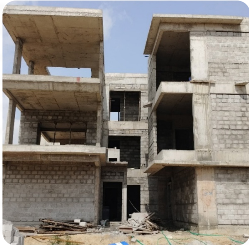
VILLA NO: 79 (Structure Completed)
