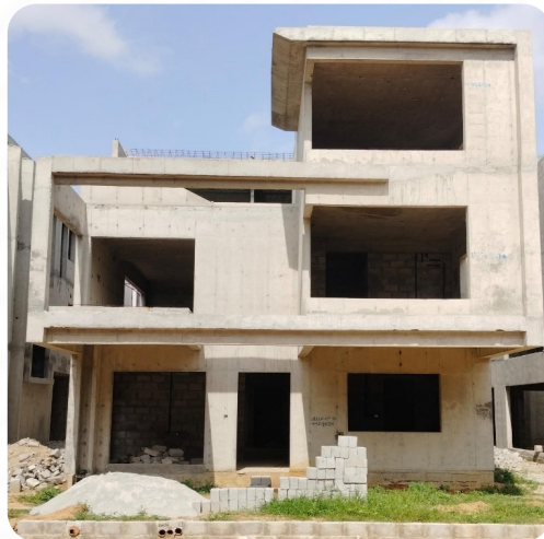
VILLA NO: 84 (Structure Completed)
