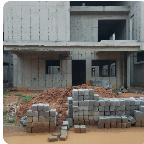
VILLA NO: 105 (Structure Completed)
