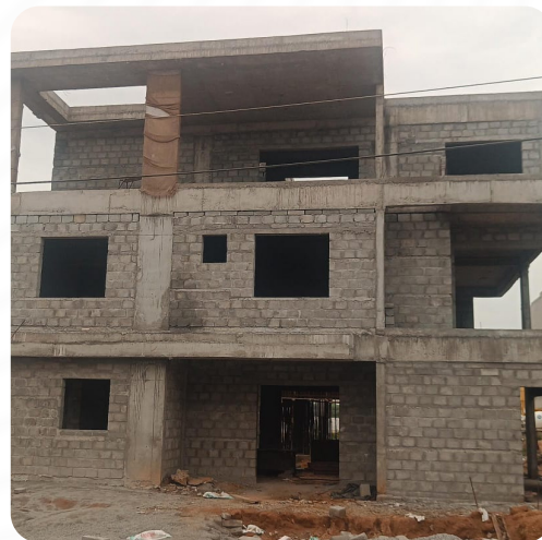
VILLA NO: 132 (Structure Completed)
