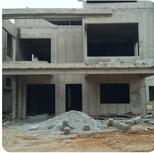
VILLA NO: 152 (Structure Completed)
