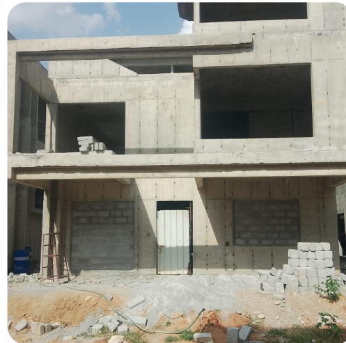
VILLA NO: 173 (Structure Completed)
