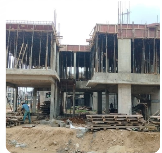
VILLA NO: 146 (FF Columns Completed)
