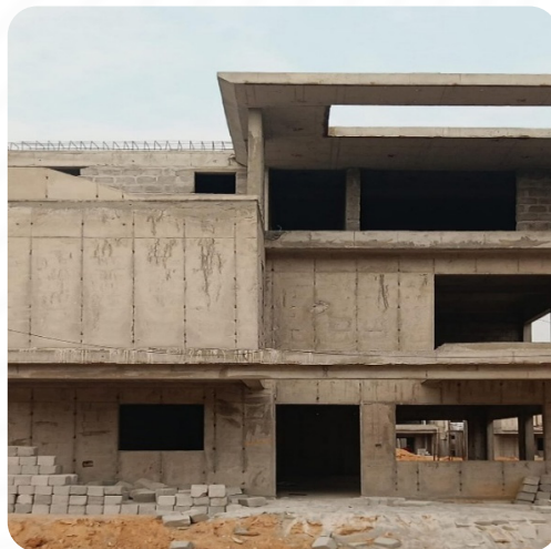
VILLA NO: 124 (Structure Completed)
