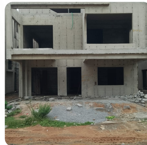
VILLA NO: 118 (Structure Completed)
