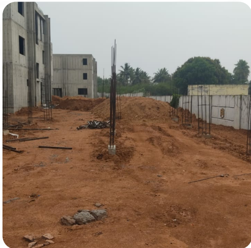
VILLA NO: 179 (Pedestals Completed)
