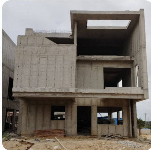
VILLA NO: 30 (Structure Completed)
