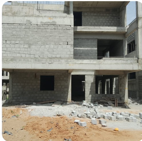
VILLA NO: 38 (Structure Completed)
