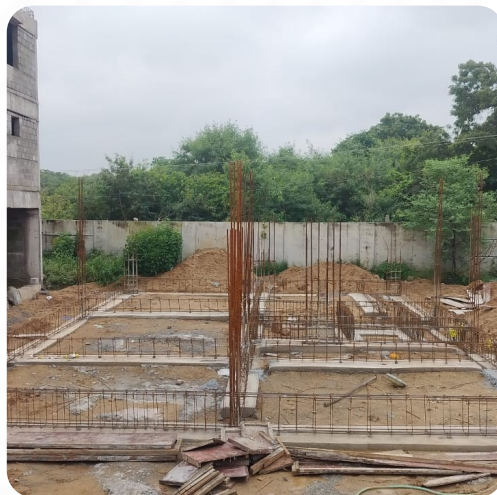
VILLA NO: 59 (Backfilling Completed)
