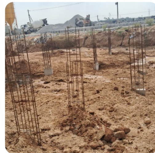
VILLA NO: 166 (Pedestals Completed)
