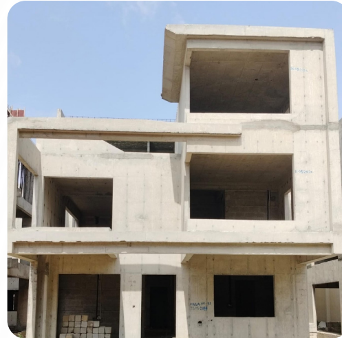
VILLA NO: 81 (Structure Completed)
