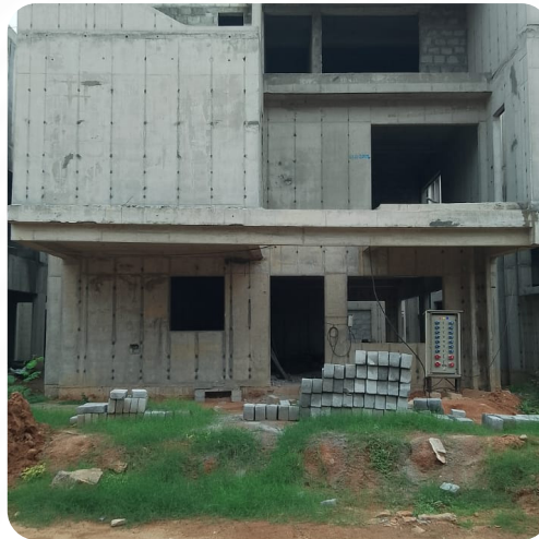
VILLA NO: 104 (Structure Completed)
