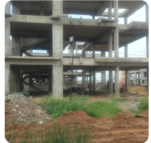
VILLA NO: 15 (SF Slab Completed)
