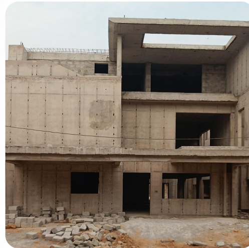
VILLA NO: 129 (Structure Completed)
