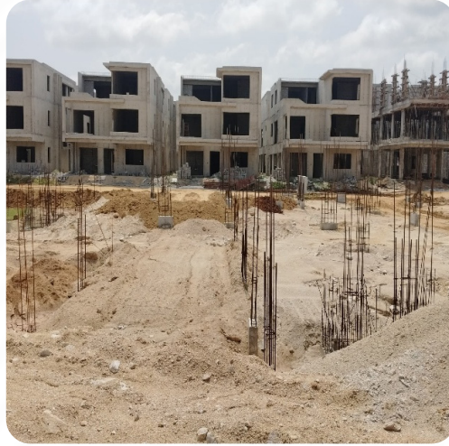
VILLA NO: 168 (Pedestals Completed)
