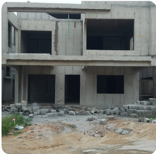
VILLA NO: 119 (Structure Completed)
