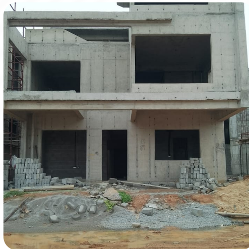
VILLA NO: 144 (Structure Completed)
