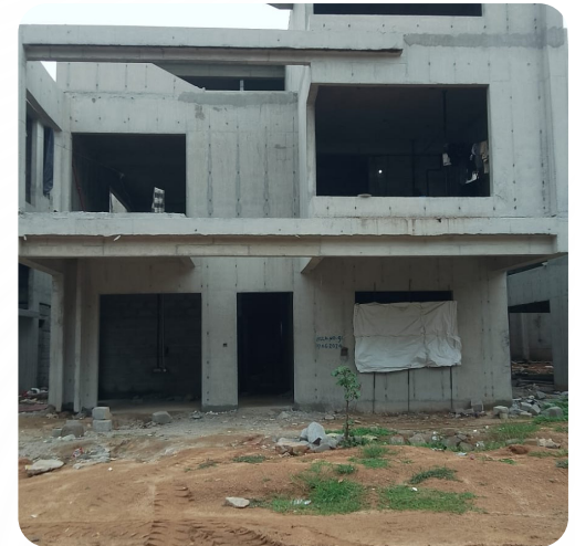
VILLA NO: 90 (Structure Completed)
