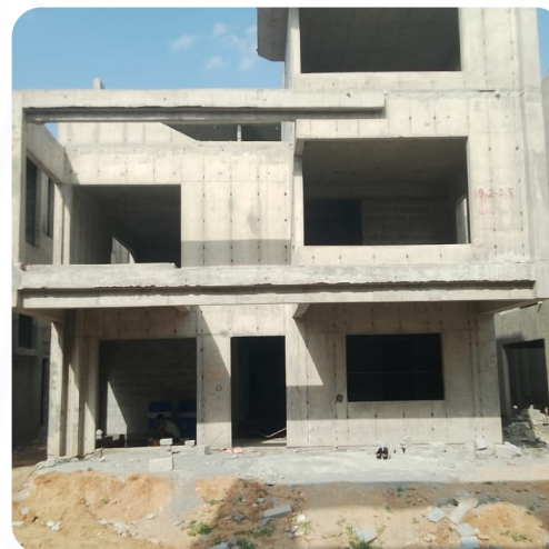
VILLA NO: 149 (Structure Completed)
