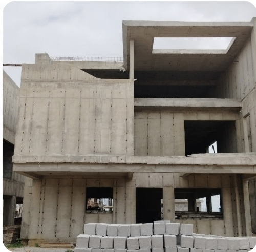
VILLA NO: 29 (Structure Completed)
