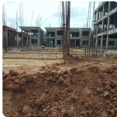
VILLA NO: 19 (Plinth Beam Completed)
