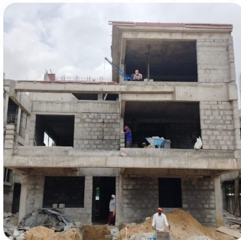
VILLA NO: 50 (Structure Completed)
