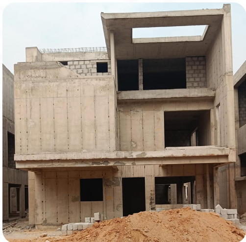
VILLA NO: 159 (Structure Completed)
