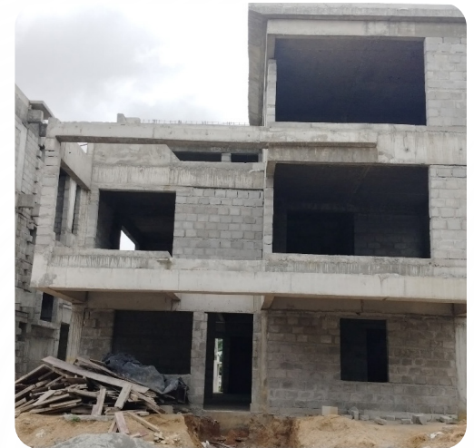
VILLA NO: 24 (Structure Completed)
