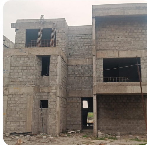
VILLA NO: 185 (Structure Completed)
