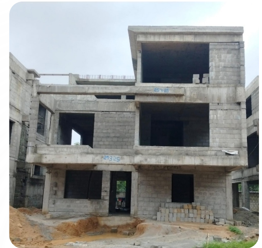
VILLA NO: 48 (Structure Completed)
