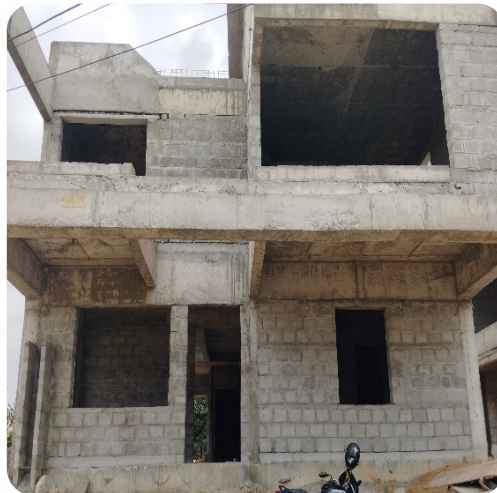
VILLA NO: 6 (Structure Completed)
