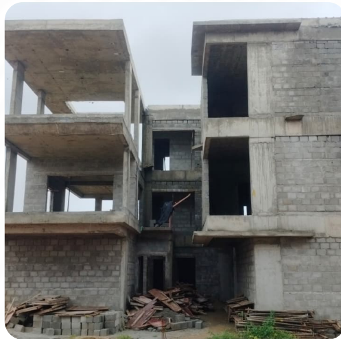
VILLA NO: 22 (Structure Completed)
