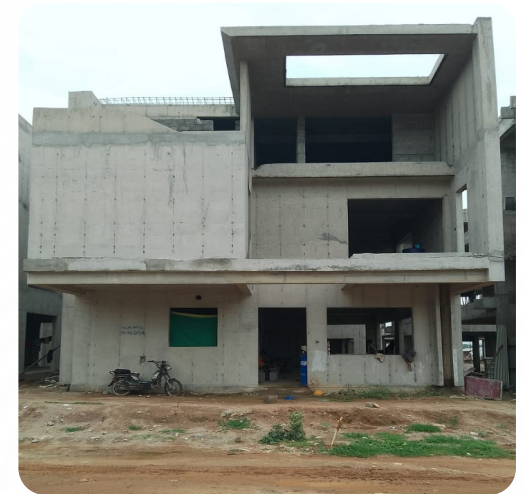
VILLA NO: 73 (Structure Completed)
