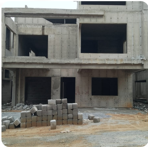
VILLA NO: 151 (Structure Completed)
