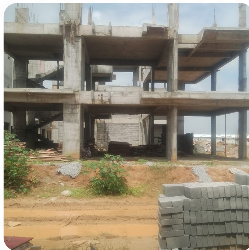
VILLA NO: 108 (SF Columns Completed)
