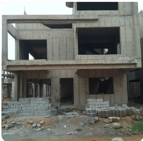
VILLA NO: 147 (Structure Completed)
