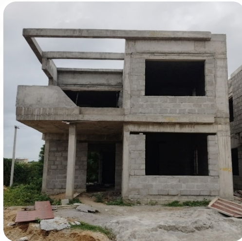
VILLA NO: 2 (Structure Completed)
