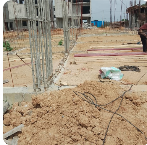
VILLA NO: 14 (Plinth Beam Completed)
