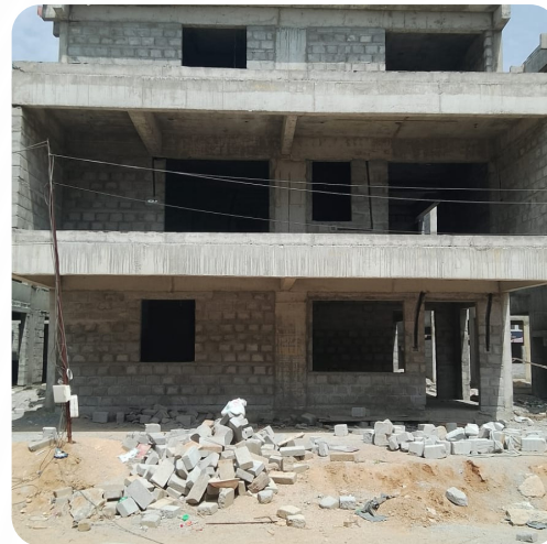
VILLA NO: 39 (Structure Completed)
