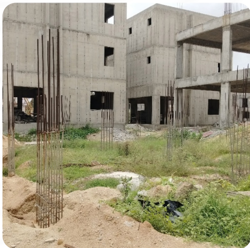
VILLA NO: 33 (Pedestals Completed)
