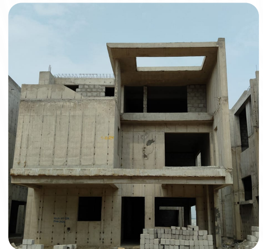
VILLA NO: 134 (Structure Completed)
