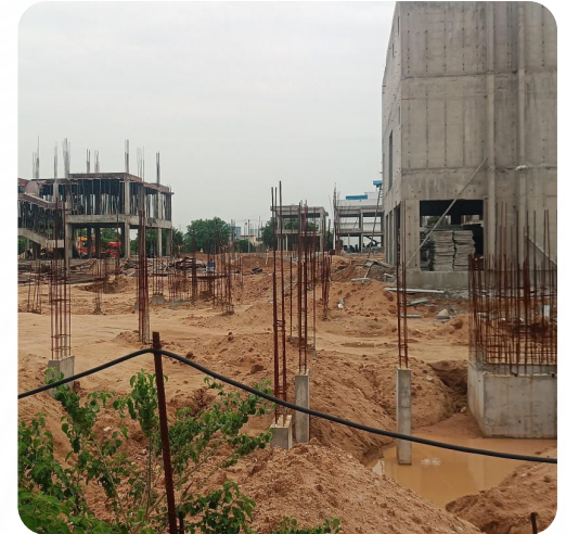
VILLA NO: 32 (Pedestals Completed)
