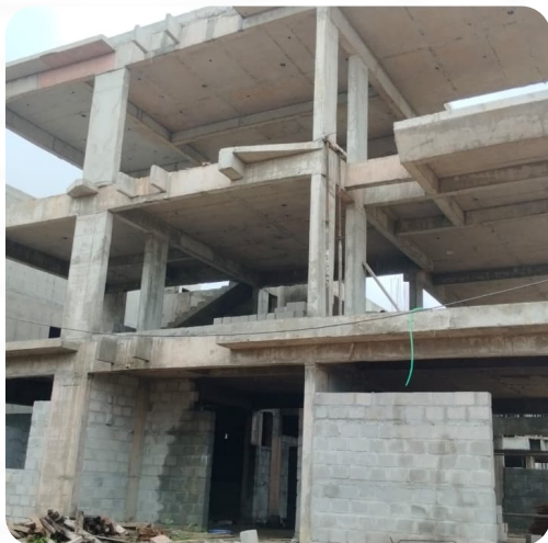
VILLA NO: 131 (SF slab Completed)
