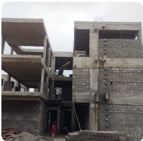
VILLA NO: 115 (Structure Completed)
