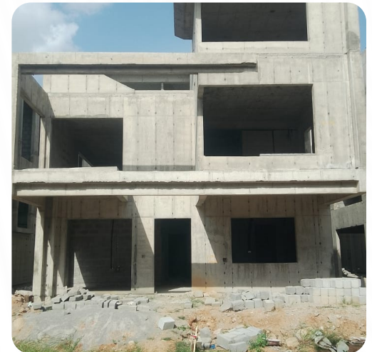
VILLA NO: 174 (Structure Completed)
