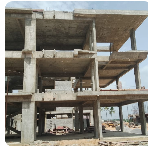
VILLA NO: 40 (Structure Completed)
