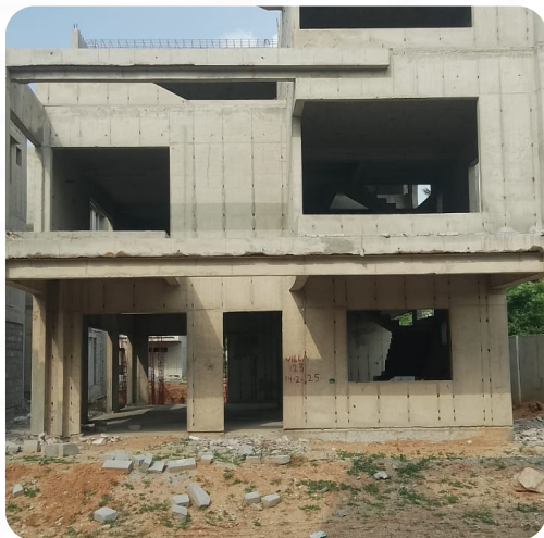
VILLA NO: 123 (Structure Completed)
