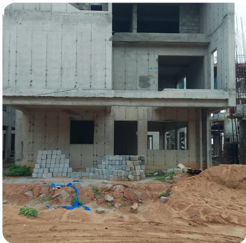
VILLA NO: 107 (Structure Completed)
