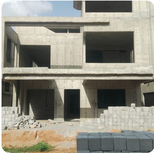
VILLA NO: 175 (Structure Completed)
