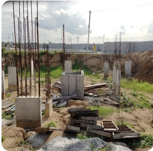
VILLA NO: 167 (Pedestals Completed)
