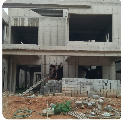
VILLA NO: 176 (Structure Completed)
