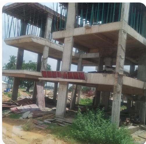
VILLA NO: 139 (SF Columns Completed)
