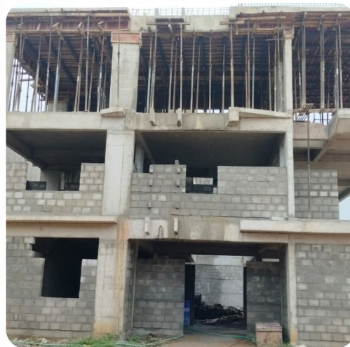
VILLA NO: 161 (SF Slab in Progress)
