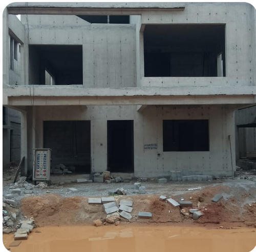
VILLA NO: 111 (Structure Completed)
