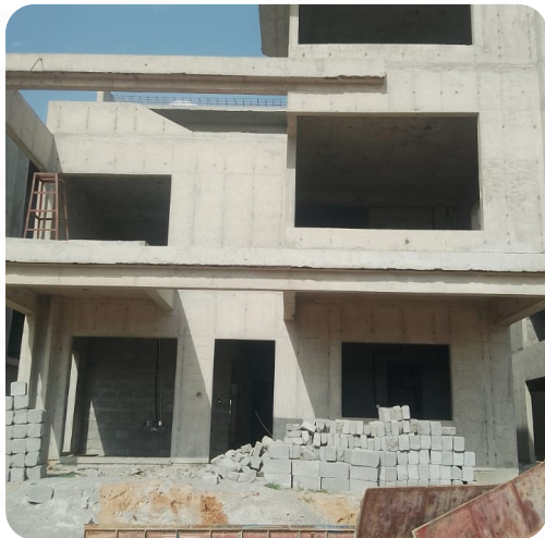
VILLA NO: 143 (Structure Completed)
