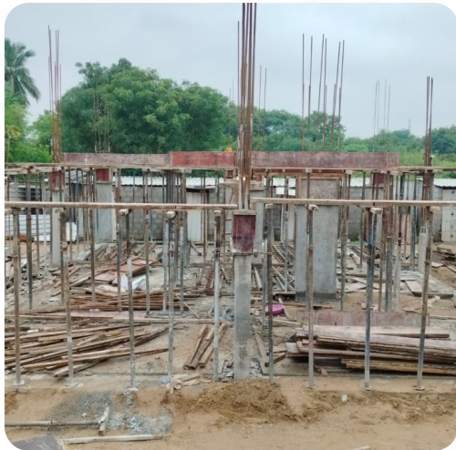
VILLA NO: 54 (GF Columns Completed)
