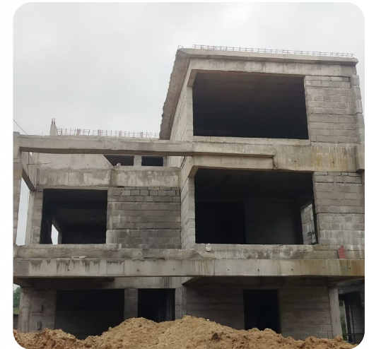
VILLA NO: 57 (Structure Completed)
