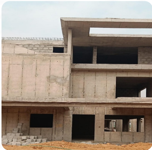
VILLA NO: 155 (Structure Completed)
