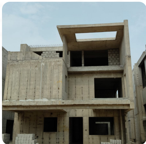
VILLA NO: 135 (Structure Completed)
