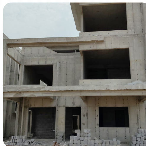
VILLA NO: 141 (Structure Completed)
