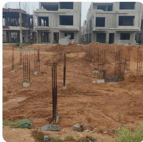
VILLA NO: 165 (Pedestals Completed)
