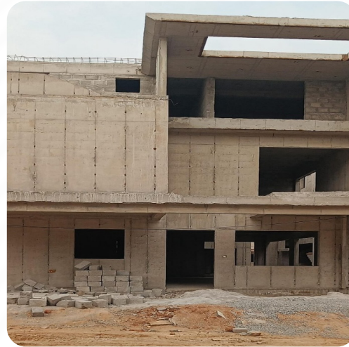
VILLA NO: 128 (Structure Completed)
