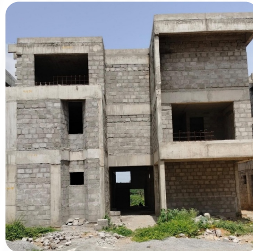
VILLA NO: 181 (Structure Completed)
