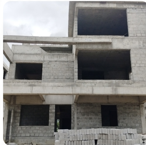
VILLA NO: 7 (Structure Completed)
