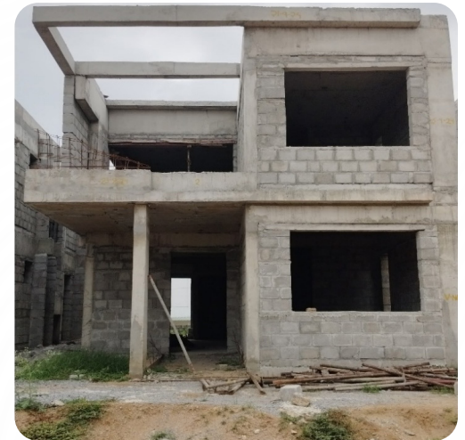
VILLA NO: 4 (Structure Completed)
