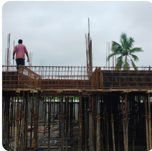
VILLA NO: 55 (GF Columns Completed)
