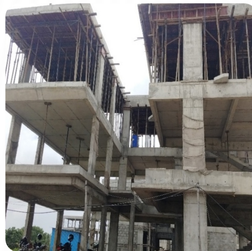
VILLA NO: 43 (SF Slab Completed)
