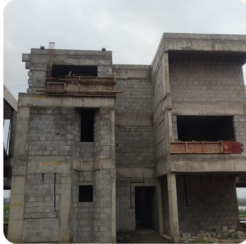
VILLA NO: 184 (Structure Completed)
