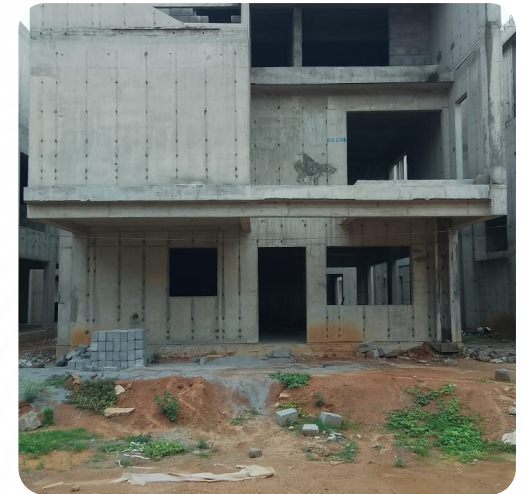
VILLA NO: 106 (Structure Completed)
