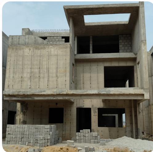
VILLA NO: 136 (Structure Completed)
