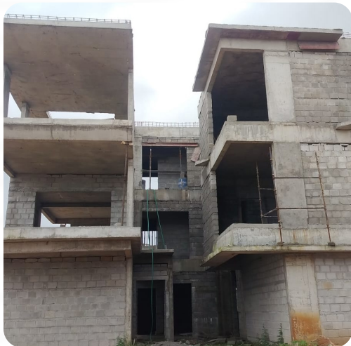
VILLA NO: 171 (Structure Completed)
