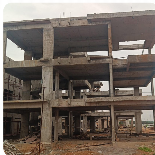
VILLA NO: 101 (Structure Completed)
