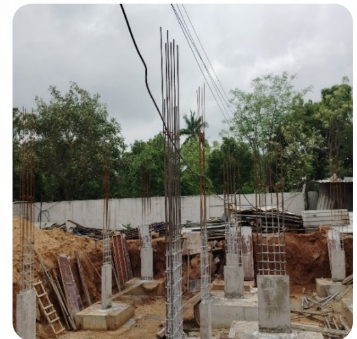
VILLA NO: 53 (Plinth Beam Completed)
