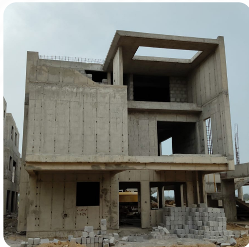
VILLA NO: 160 (Structure Completed)
