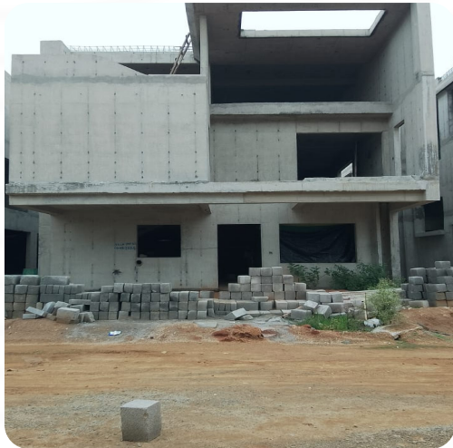
VILLA NO: 70 (Structure Completed)
