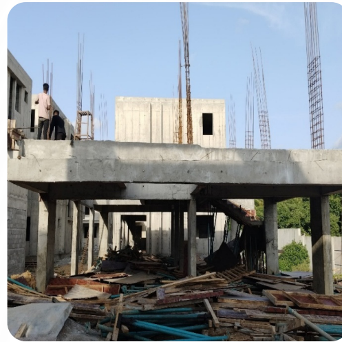
VILLA NO: 153 (GF Slab Completed)
