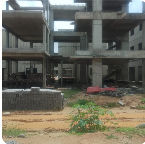
VILLA NO: 80 (Structure Completed)
