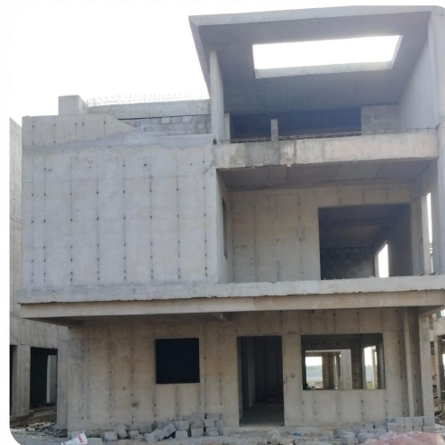
VILLA NO: 137 (Structure Completed)
