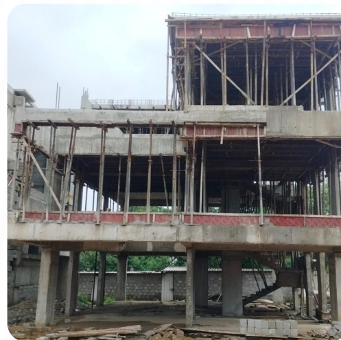
VILLA NO: 51 (SF Slab Completed)
