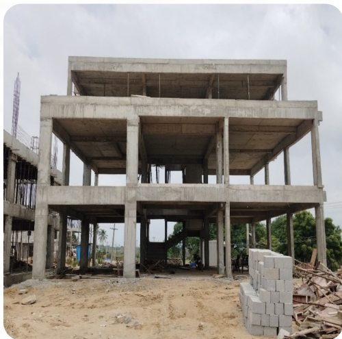
VILLA NO: 17 (SF Slab Completed)
