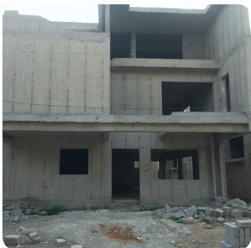
VILLA NO: 99 (Structure Completed)
