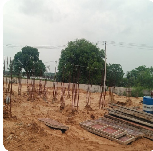
VILLA NO: 31 (Pedestals Completed)
