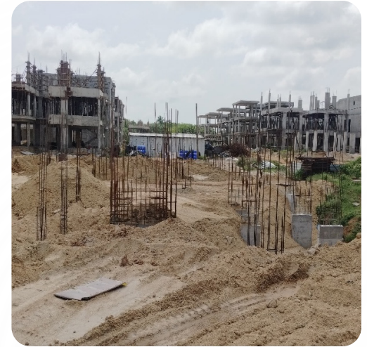
VILLA NO: 170 (Footings Completed)
