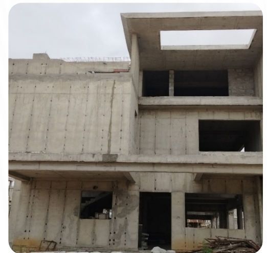
VILLA NO: 28 (Structure Completed)
