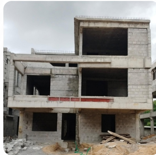
VILLA NO: 47 (Structure Completed)
