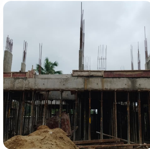
VILLA NO: 56 (FF Columns Completed)
