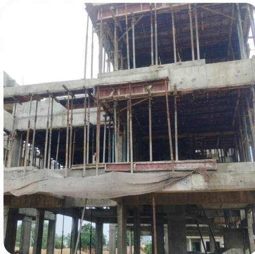
VILLA NO: 18 (SF Slab Completed)
