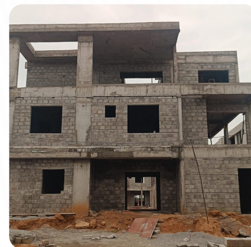
VILLA NO: 102 (Structure Completed)
