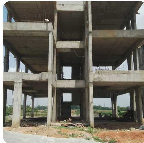
VILLA NO: 180 (Structure Completed)
