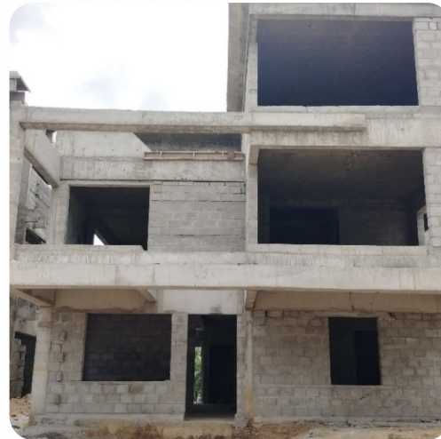
VILLA NO: 23 (Structure Completed)
