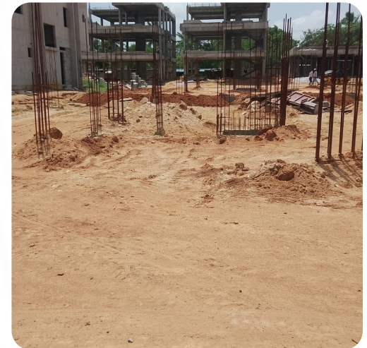
VILLA NO: 86 (Back Filling Completed)
