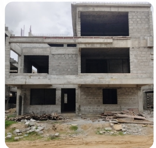
VILLA NO: 36 (Structure Completed)
