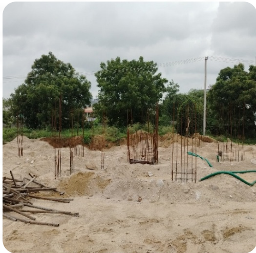
VILLA NO: 1 (Pedestals Completed)
