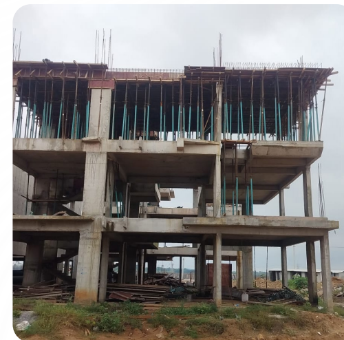
VILLA NO: 138 (SF Columns Completed)
