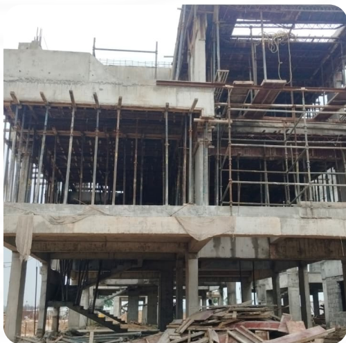
VILLA NO: 41 (Structure Completed)
