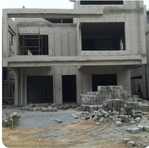
VILLA NO: 120 (Structure Completed)
