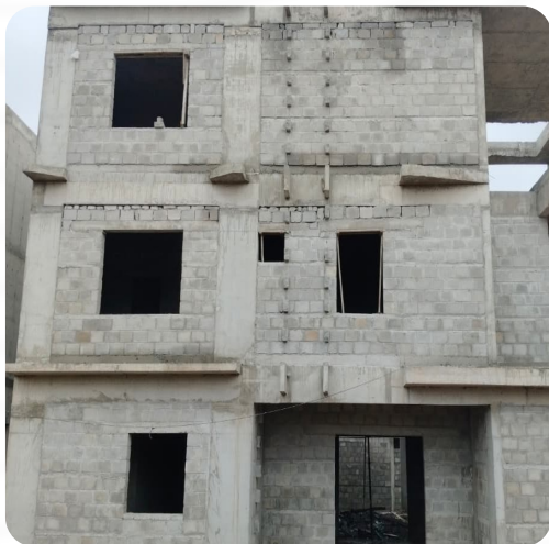
VILLA NO: 74 (Structure Completed)
