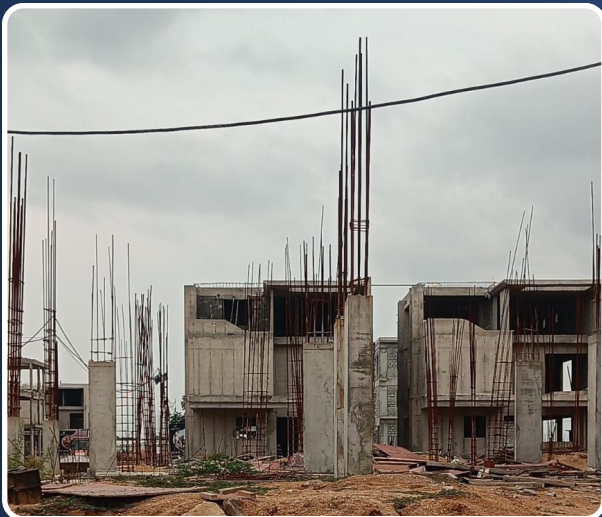
VILLA-12 (Ground Floor Columns Completed)
