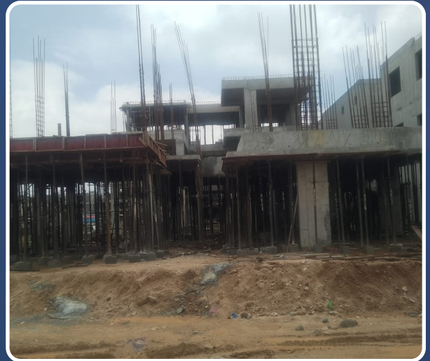
VILLA-146 (GF Slab Completed)
