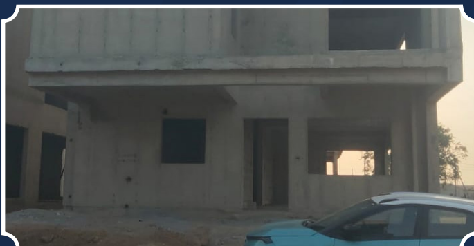
VILLA-76 (Parapet RCC Completed)
