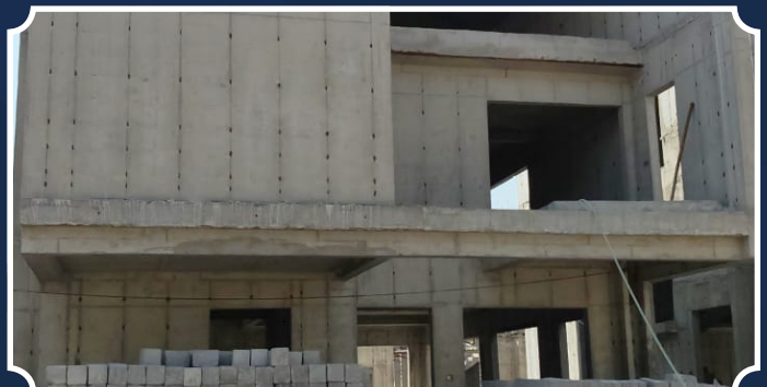
VILLA-126 (SF Slab RCC Completed)
