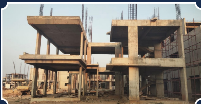
VILLA-117 (Parapet RCC Completed)
