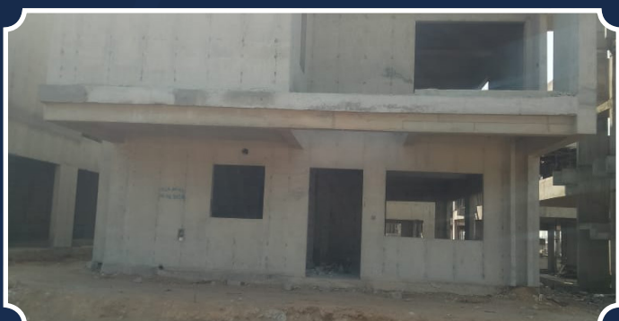
VILLA-65 (Parapet RCC Completed)
