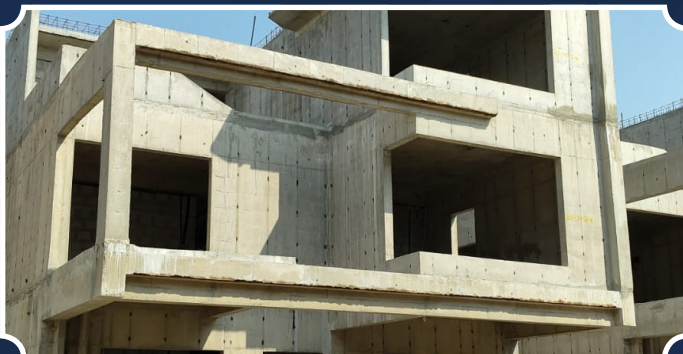
VILLA-119 (Parapet RCC Completed)
