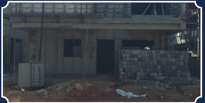
VILLA-100 (GF Slab RCC Completed)
