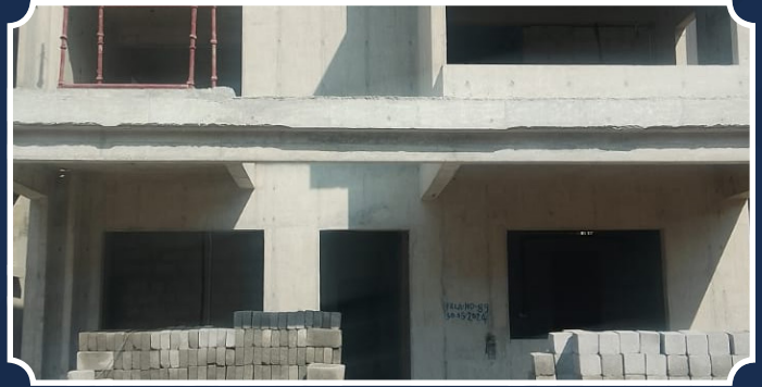
VILLA-89 (Parapet RCC Completed)
