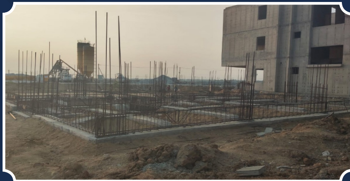
VILLA-145 (Plinth beam RCC inprogress)
