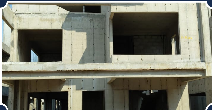
VILLA-117 (Parapet RCC Completed)
