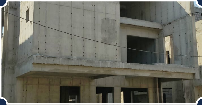
VILLA-129 (SF Slab RCC Completed)
