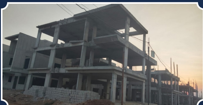
VILLA-66 (Parapet RCC Completed)
