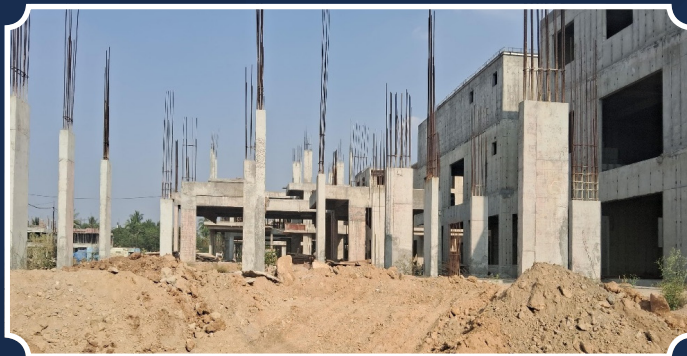
VILLA-146 (GF Columns/Walls RCC Completed)
