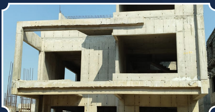
VILLA-147 (Parapet RCC Completed)
