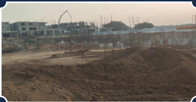
VILLA-164 (Villa Backfilling in progress)
