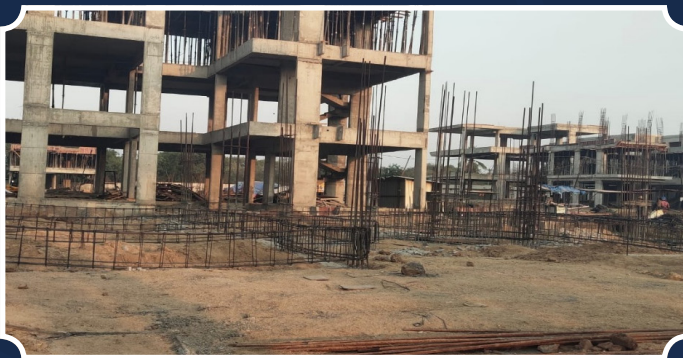
VILLA-115 (Plinth beam RCC In progress)
