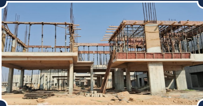
VILLA-139 (FF Slab RCC in progress)
