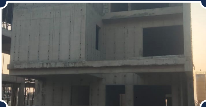
VILLA-133 (Parapet RCC Completed)
