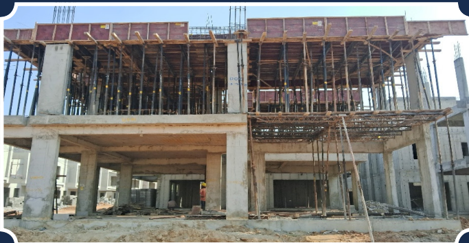
VILLA-101 (FF Columns RCC Completed)
