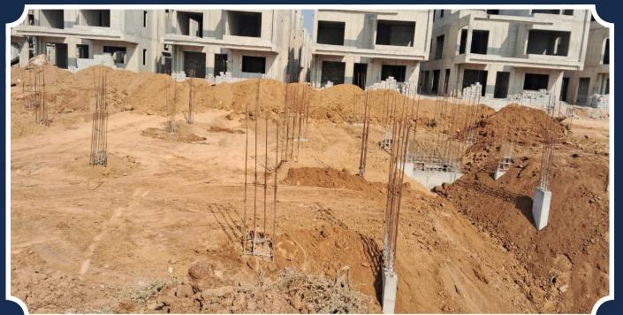
VILLA-165 (Villa Backfilling in progress)
