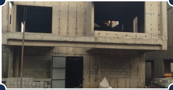
VILLA-113 (Parapet RCC Completed)
