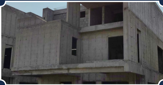
VILLA-156 (Parapet RCC Completed)
