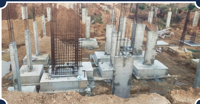
VILLA-168 (Pedastal RCC in progress)
