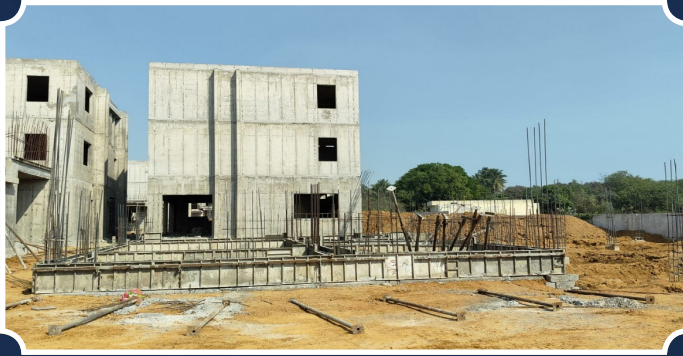
VILLA-178 (Plinth Beam PCC in progress)
