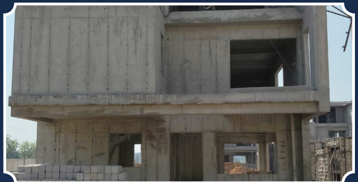
VILLA-124 (Parapet RCC Completed)
