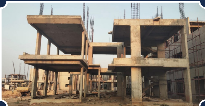
VILLA-109 (FF Slab RCC Completed)
