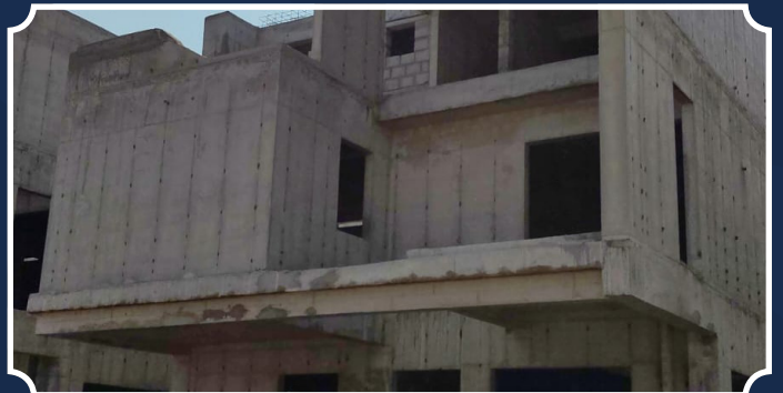
VILLA-159 (Parapet RCC Completed)
