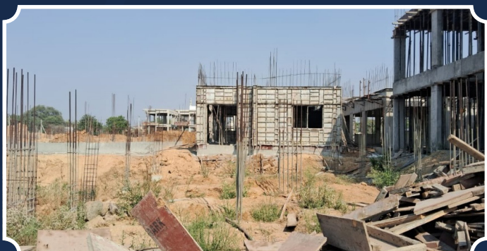
VILLA-33 (Villa backfilling in progress)
