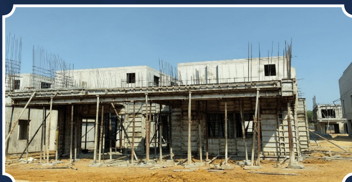
VILLA-152 (GF Slab RCC in progress)
