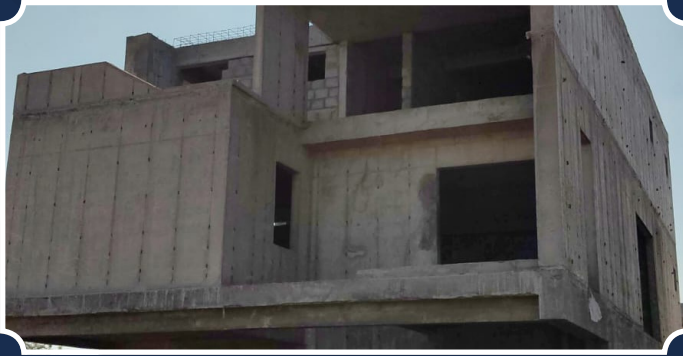
VILLA-154 (Parapet RCC Completed)
