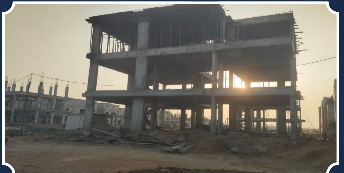
VILLA-102 (SF Slab RCC Completed)
