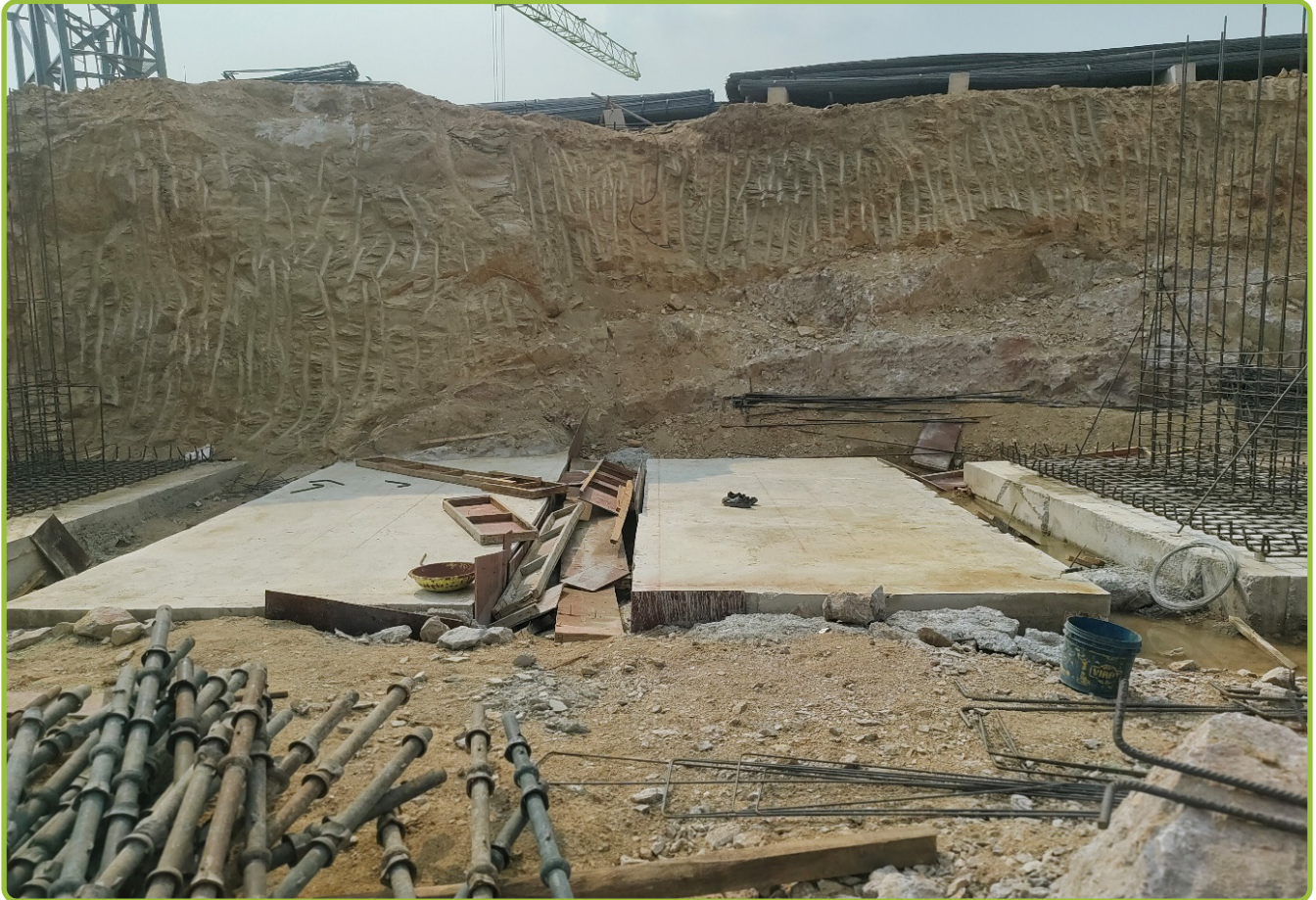
Tower-D PCC for Footings is in progress
