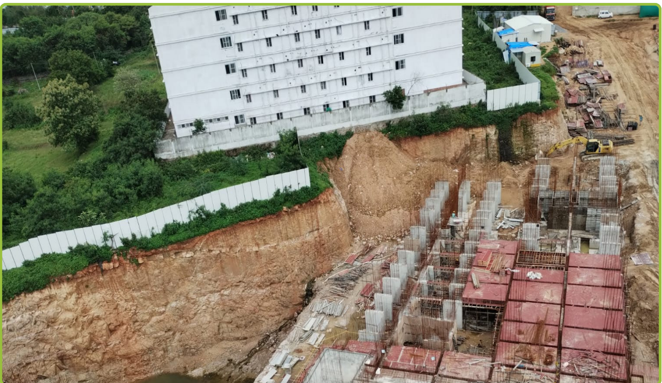
Tower-B (BASEMENT 2 CASTING)
