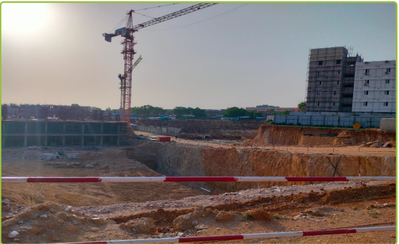
Tower-A Excavation Completed
