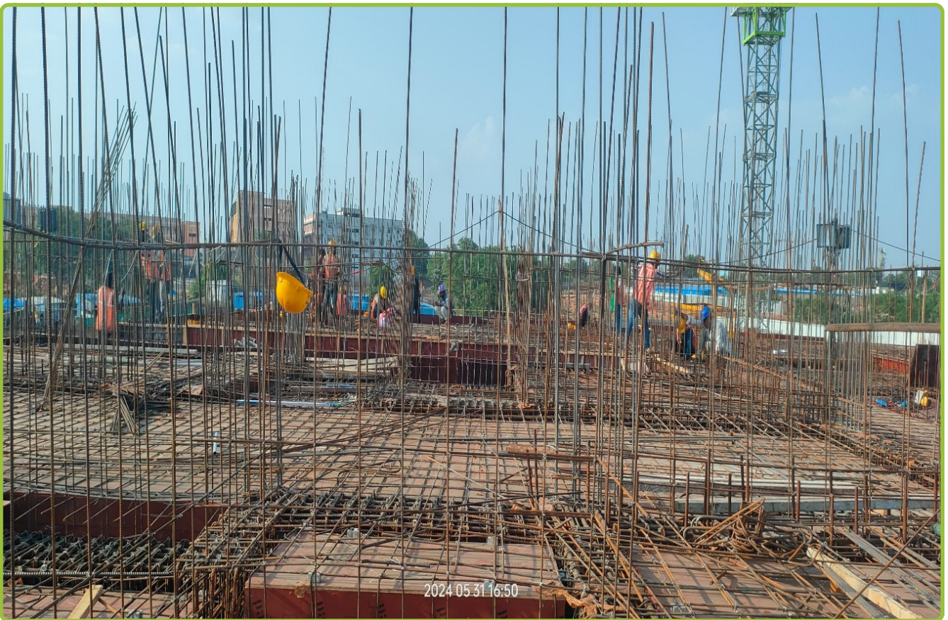
Tower-C Ground Level Slab Work
