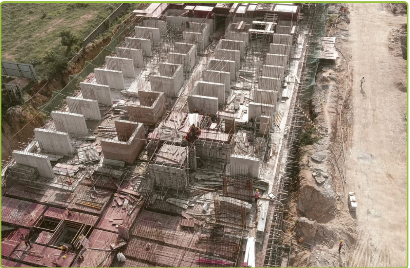
Tower-B Footings Completed
