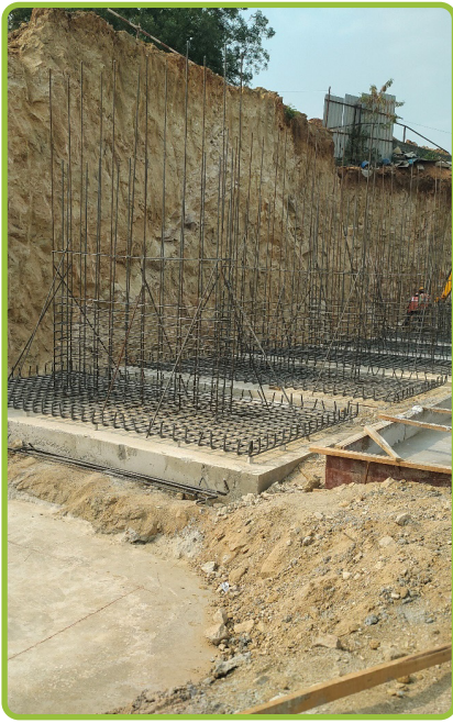
Tower-D Footings Reinforcement work is in progress
