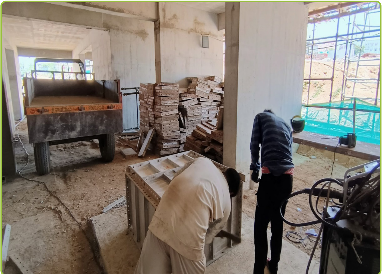
I Form fabrication yard & Mivan shuttering boards making work in progress
